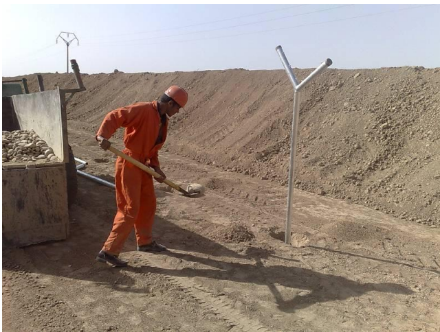
Site Photo 5. Installing posts for the PEZ fence post (Photo courtesy of the USACE)
