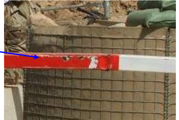
Site Photo 16. Close-up of Site Photo 15
