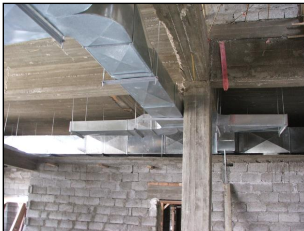
Poor concrete work and ductwork at the Hai Alasra Wa Al Mafqodeen Primary Health Care Center
