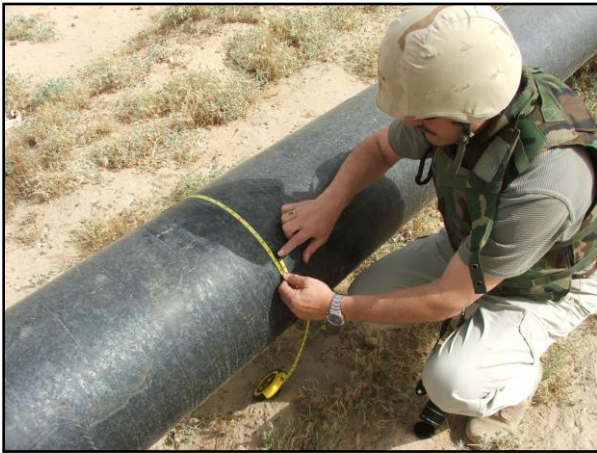
Inspector measuring pipe diameter
