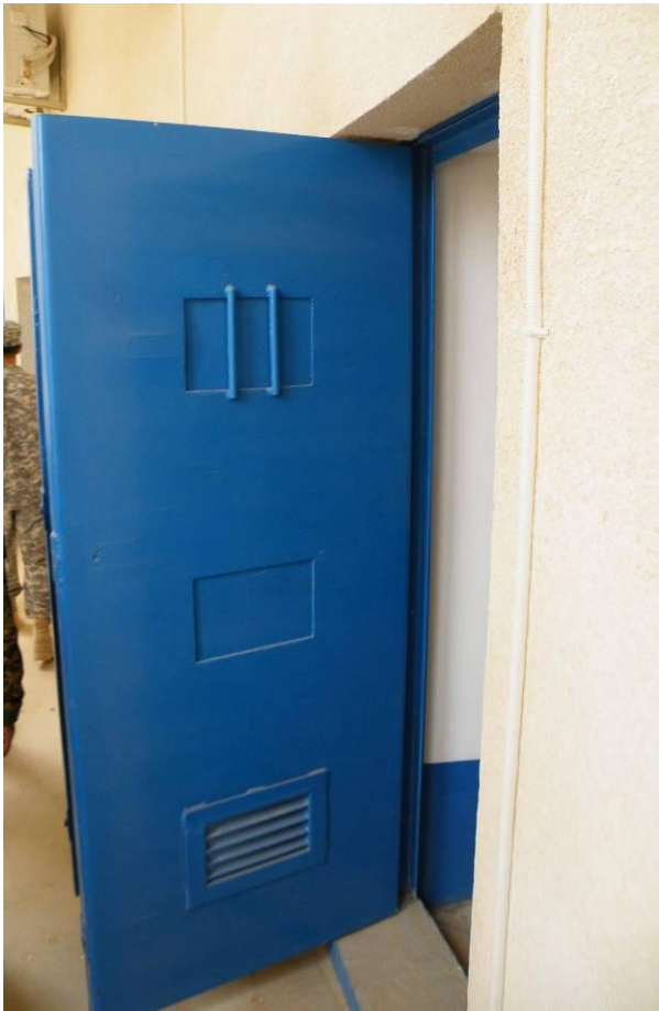
Site Photo 16. Steel prison cell door
