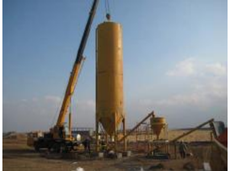
Site Photo 4. Installation of on-site batch plant (Courtesy of USACE)
