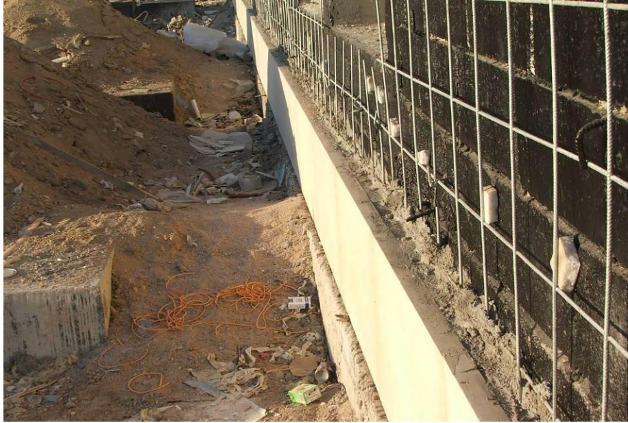
Site Photo 4. Exterior stone cladding installation
