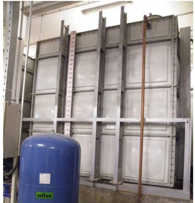
Site Photos 19 and 20. Water booster pumps and storage tanks
