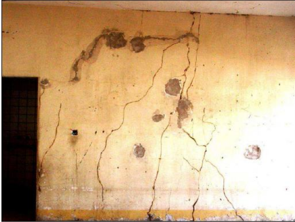
Photo 1. Termite tubes in a concrete structure in Basrah, Iraq (Courtesy of GRS)
