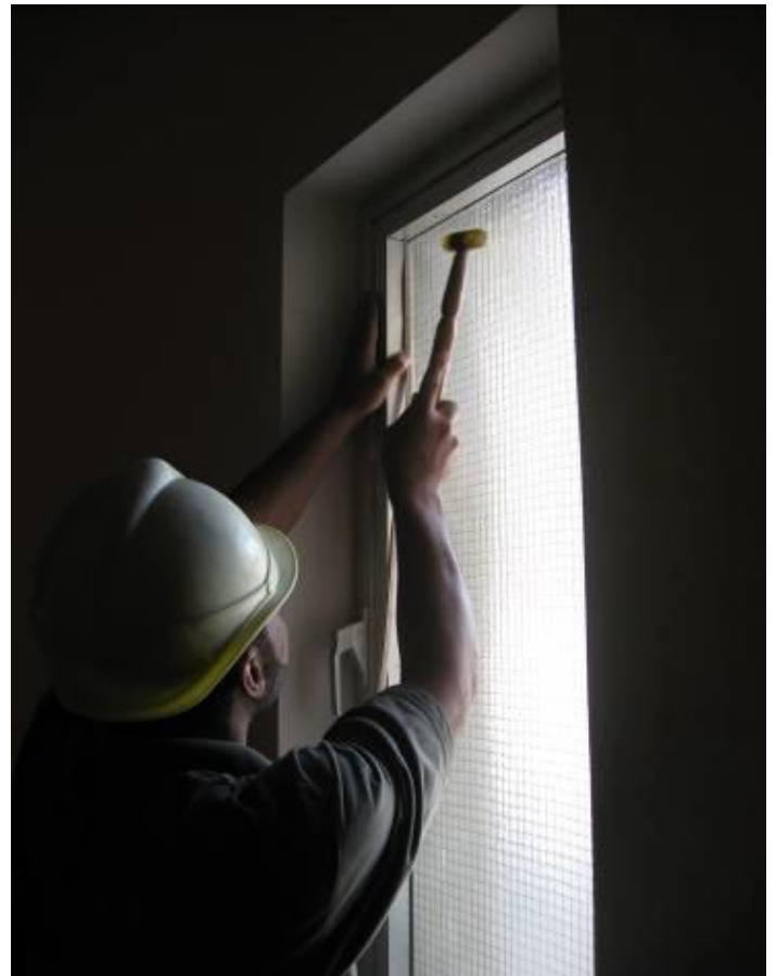
Site Photo 6. Installation of ballistic glass for windows
