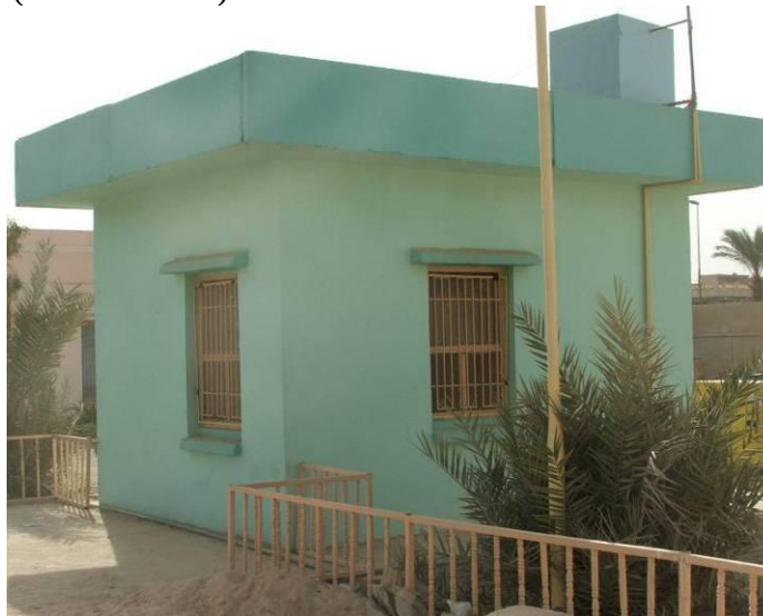
Site Photo 30. Caretaker building (Al Faoo)
