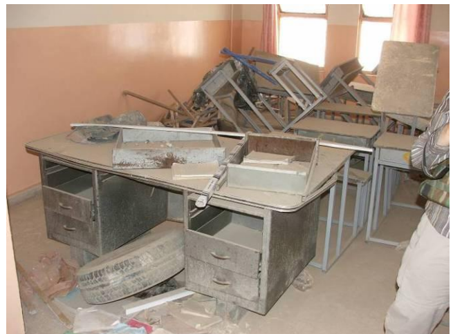
Site Photo 44. Unfinished 2 nd floor (Al Faoo)
