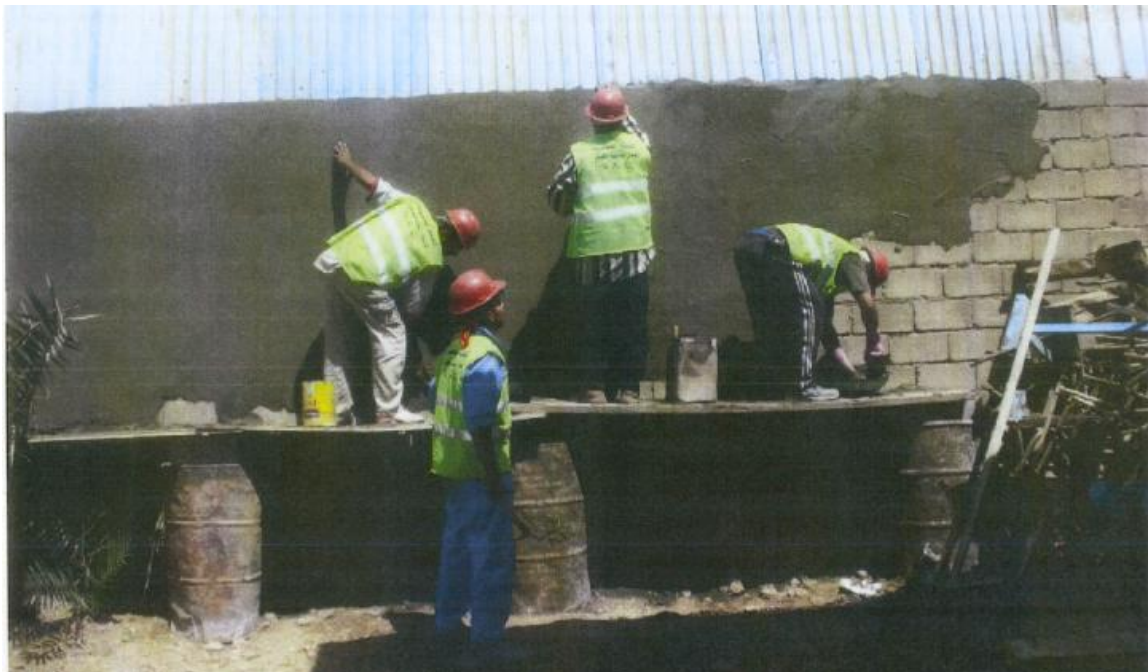
Site Photo 5. Plastering the wall at Al Mualameen (Photo courtesy of MNC-I)
