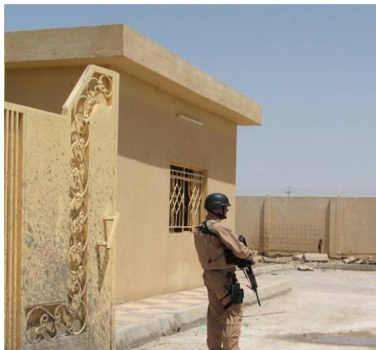
Site Photo 9. Operator building
