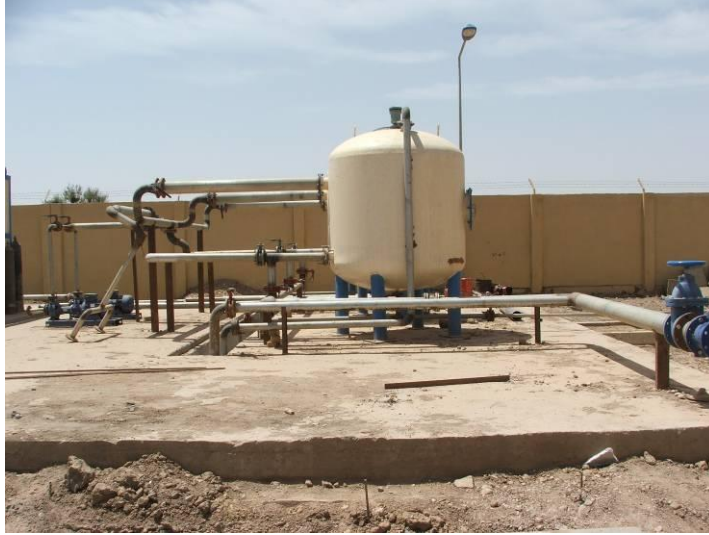
Site Photo 5. Reinforced concrete pad for 50-m 3 /hr compact unit water treatment plant
