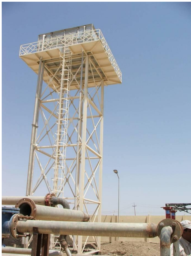
Site Photo 13. Elevated storage tank
