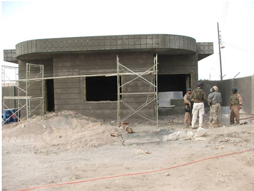
Site Photo 6. Operator building
