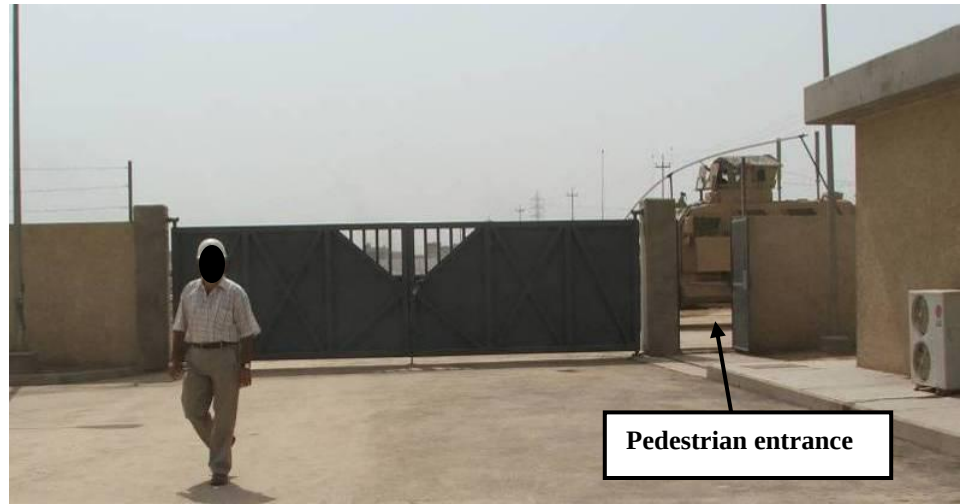
Site Photo 4. Perimeter gate (with pedestrian entrance)
