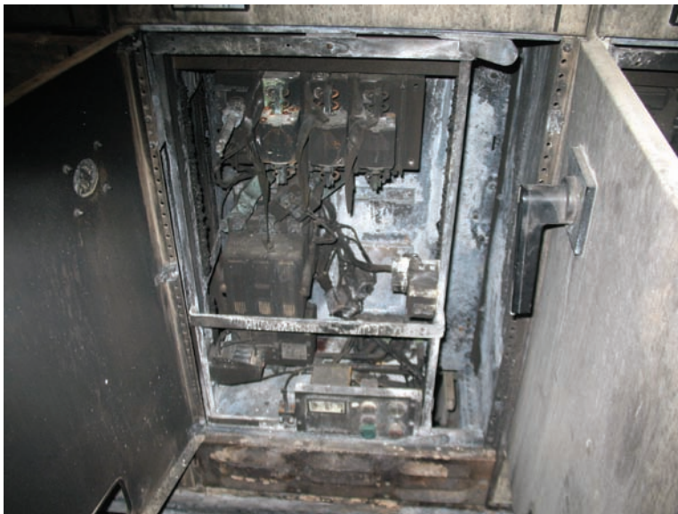
Burnt wiring in the control center at the Doura Power Station. The fire resulted from exciter flashover caused by repeated "hard tripping."
