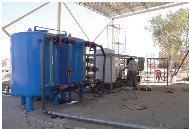
Reverse osmosis unit at installation (contractor-provided photo).
