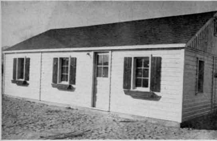
Completed Prefabricated House. Four days—31½ Hours after arrival of materials.
