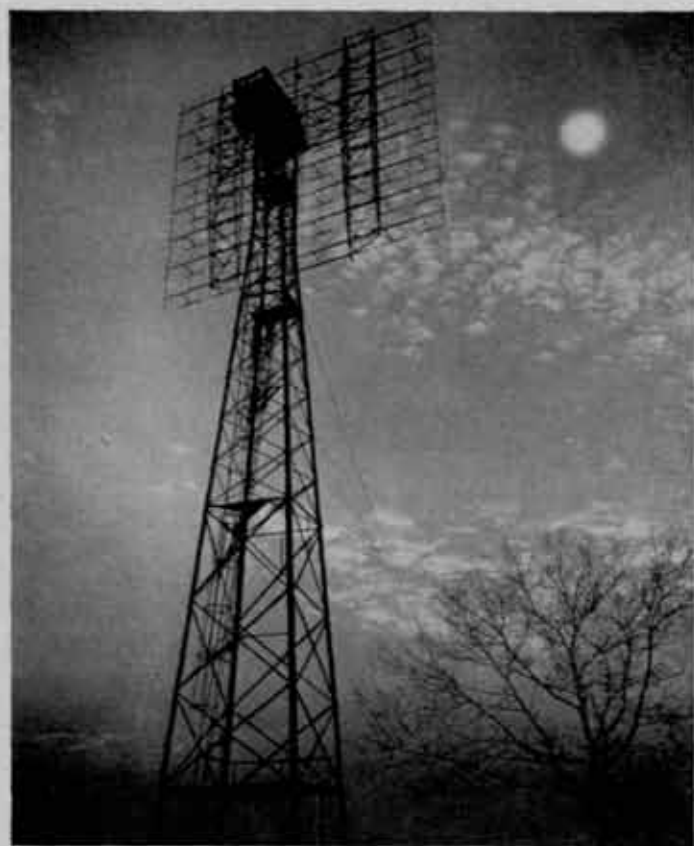
In contrast to the earlier sets, here is a picture of the Radar Antenna used by the Signal Corps in making first contact with the moon in January 1946.
