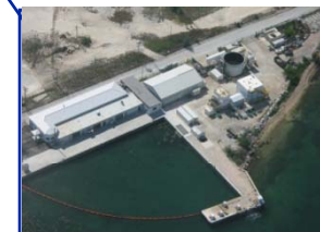
KEY WEST Marine Corrosion Facility
