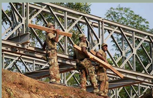
Providing Exercise Related Construction (ERC)
