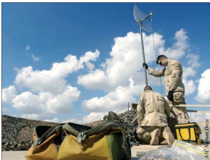
Figure 2. SrA Ricardo Reveles and AIC Sven Bickham install an antenna and align a satellite dish for the best signal.
