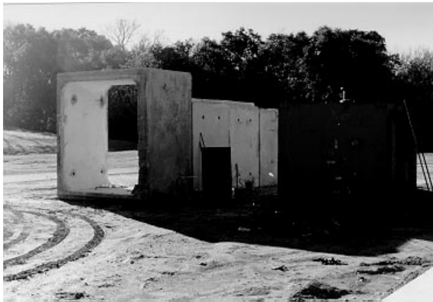
Figure 2.5 Photo Showing Concrete Reflecting Walls Opposite Blast Chamber
