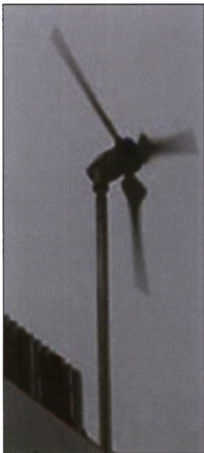
Mr. Boswell's B1500, which produces nearly 30,000 Watts, stands 20-30 feet tall on a 3-foot by 2-foot deep concrete pad.
