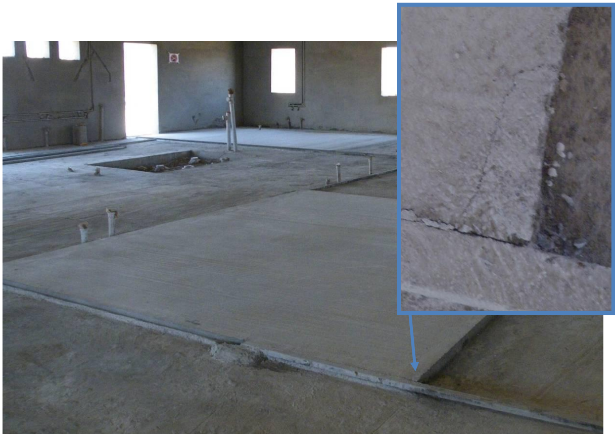
Site Photo 8. Construction of mortar overlay on floor slab.
