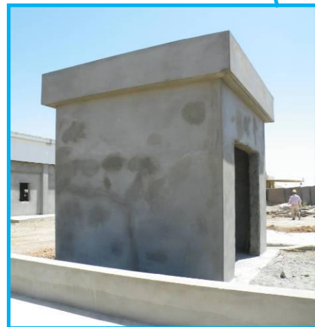
Site Photo 4. Pump room
