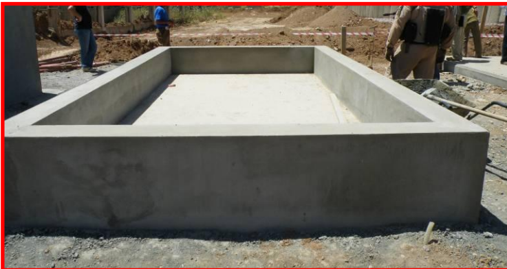
Site Photo 3. Fuel tank base
