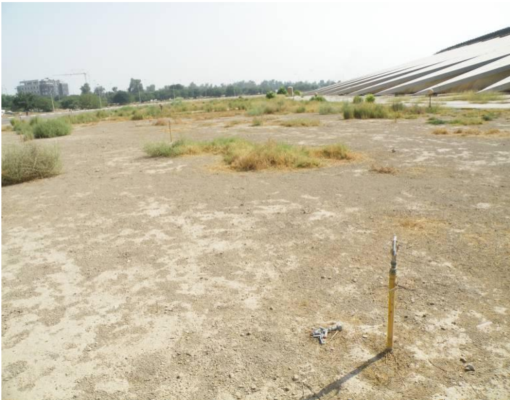
Site Photo 10. Sprinkler heads
