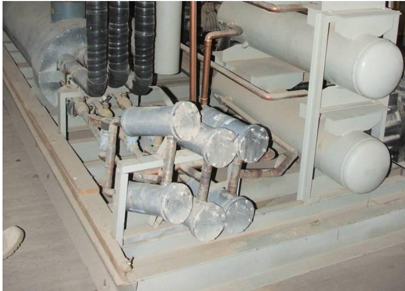
Site Photo 16. Damaged dairy production equipment
