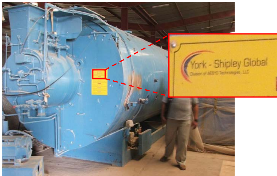
Site Photo 17. Dairy production equipment
