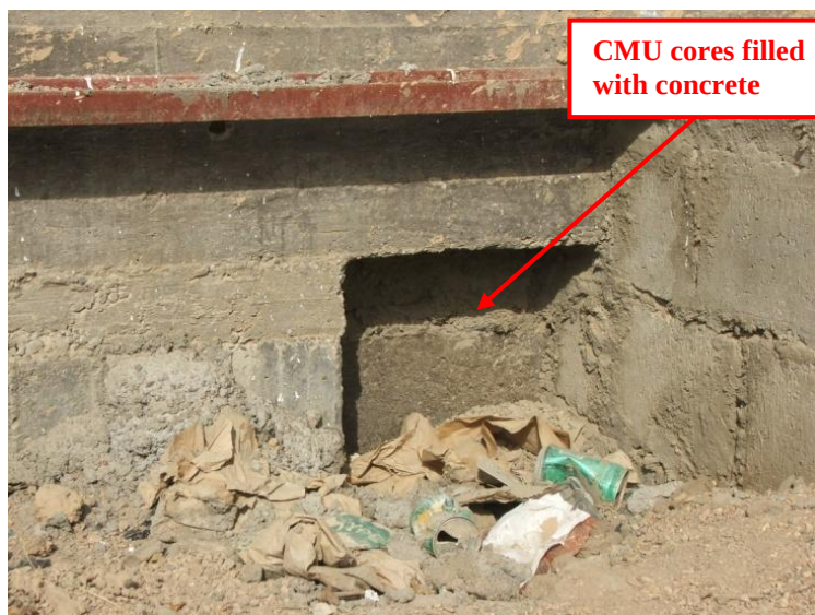
Site Photo 23. CMU cores filled with concrete
