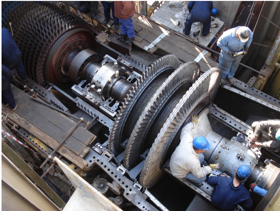
Figure 3—Turbine Generator under Repair
