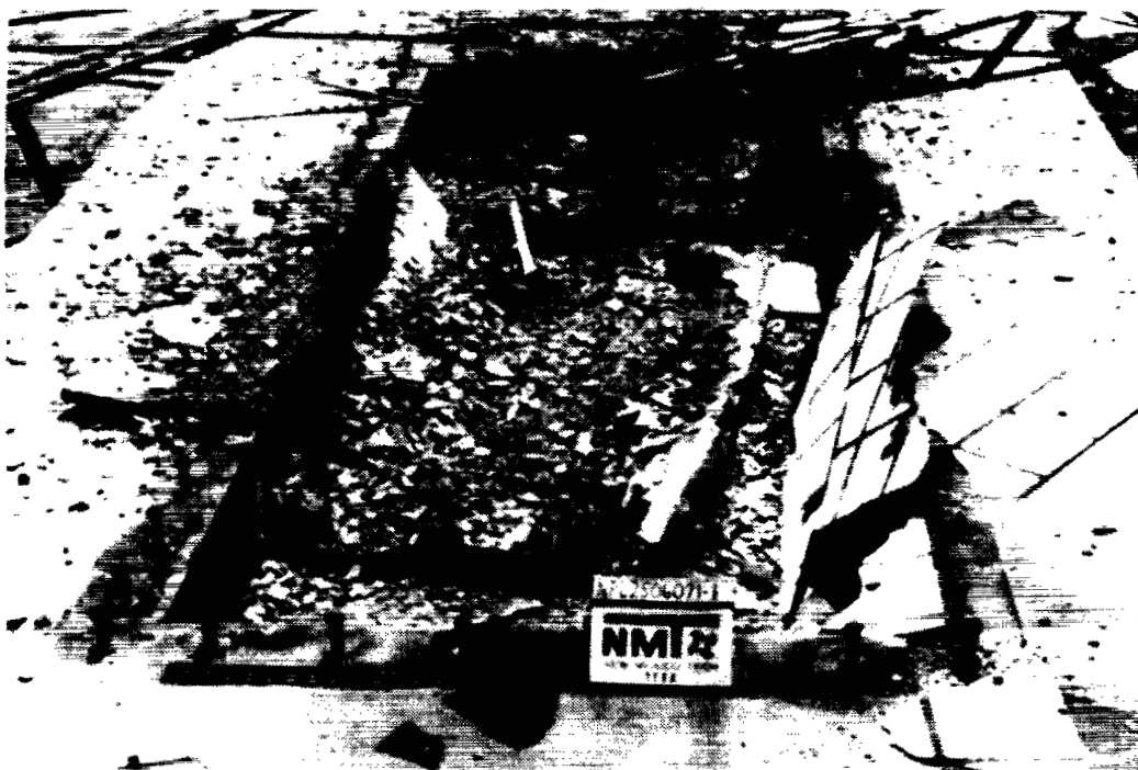
Figure 11. Post-test overall view of Test 1 roof.
