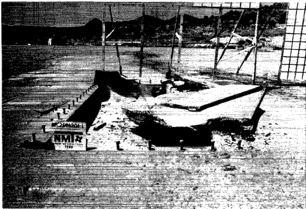
Figure 13. Post-test overall view of Test 2 roof.
