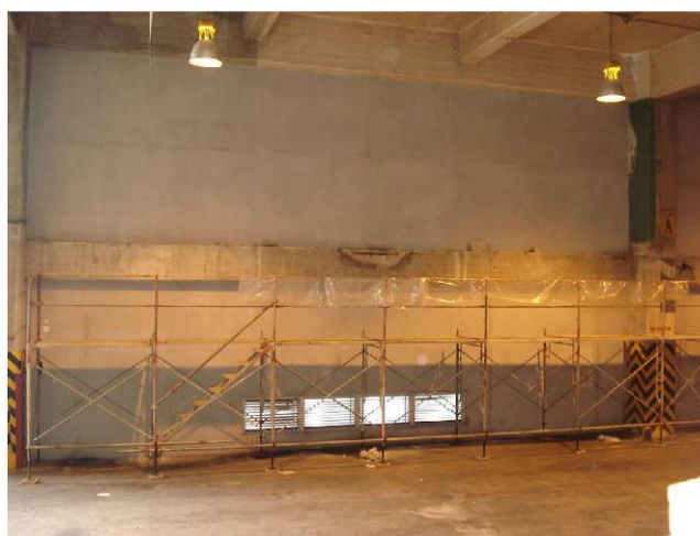
Figure 15. Overview of “Beam 1” at Naha Port Building 306.
