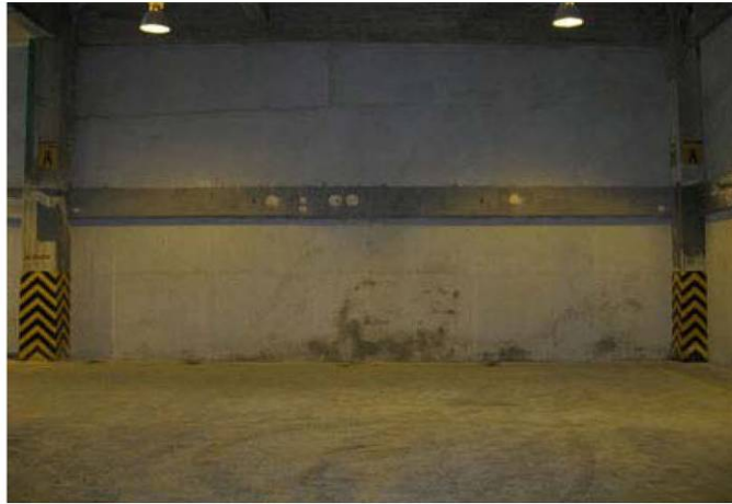
Figure 1g. Overall view of beam “A” after treatment; reportedly a zinc-aluminum-indium rich coating was applied to the concrete beam surface
