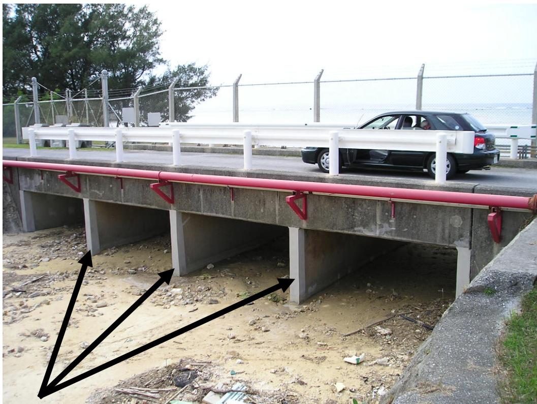
Figure 2.4. Tank farm culvert 3, vertical concrete support components.
