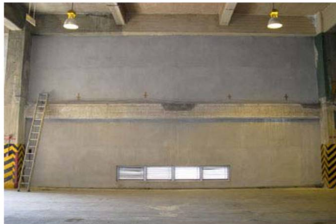
Figure 1f. Overall view of beam "AA" after treatment; reportedly treatment consisted of vapor and liquid inhibitor application to the concrete beam surface
