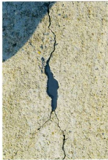
CHEMPRON APPLICATION AT SETHOUR JOHNSON AIR FORCE BASE
