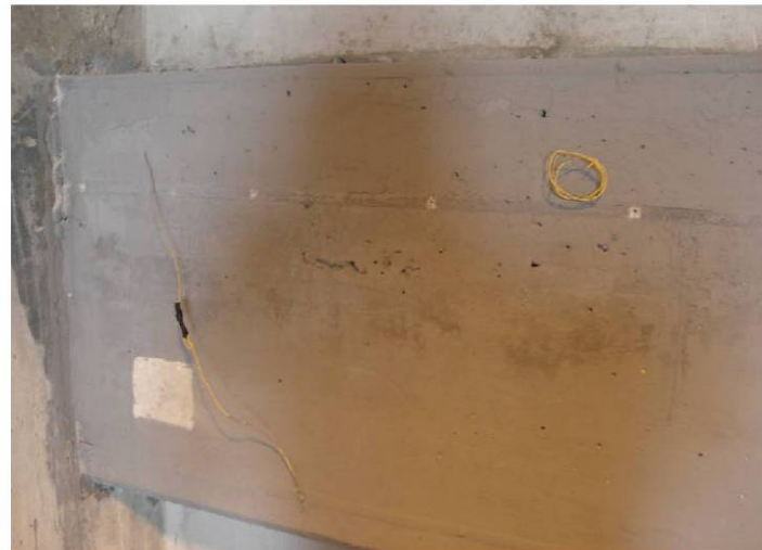
Figure 23. Close up showing titanium mesh connections in sacrificial coating.
