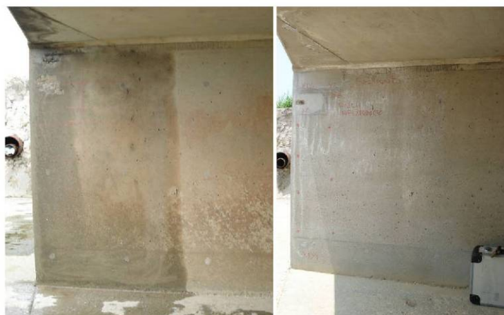
Figure 5. Typical appearance of culvert before (left) and 6 months after (right) inhibitor application.
