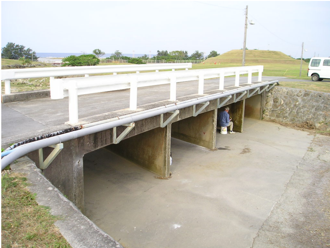
Figure 2.3. Tank farm culvert 2, all concrete surfaces.
