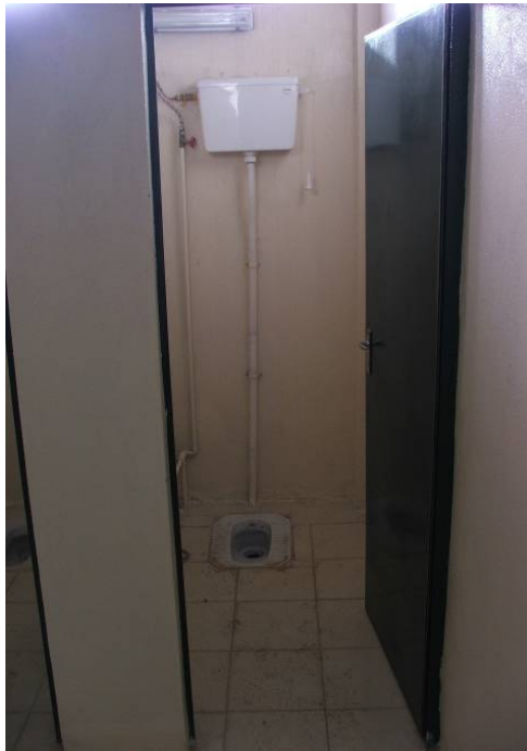
Site Photo 7. Eastern toilet in bathroom
