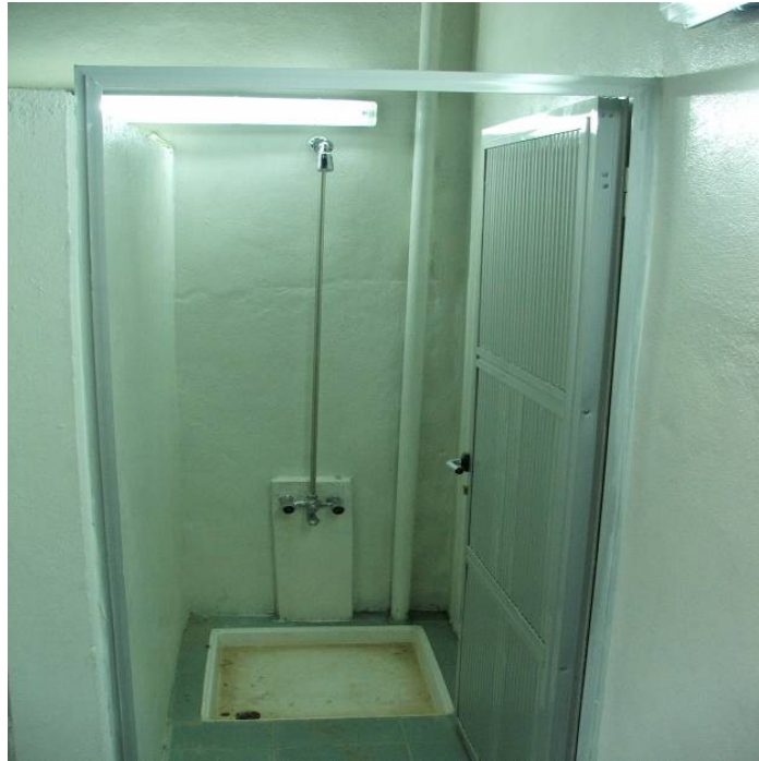
Site Photo 24. Inside of shower
