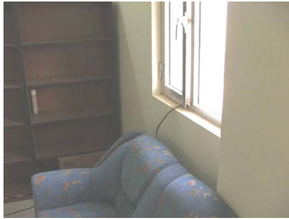
Site Photo 17. Window within the resting room
