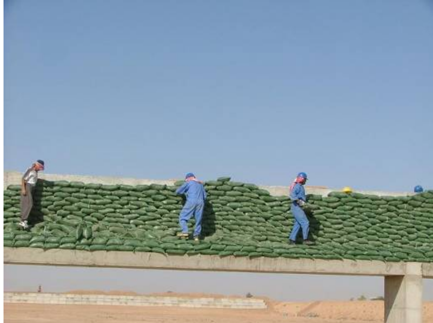
Site Photo 11. Small arms range baffle under construction (Photo courtesy of ECC)
