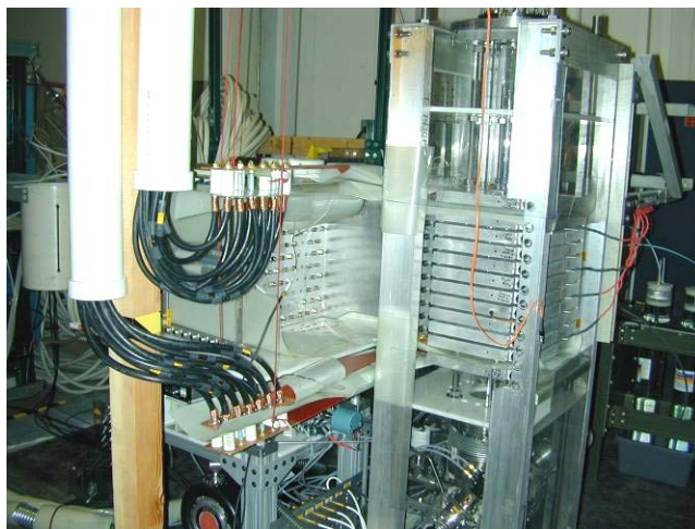
Figure 38. Cusp coil transmission-line cables and headers (center)
