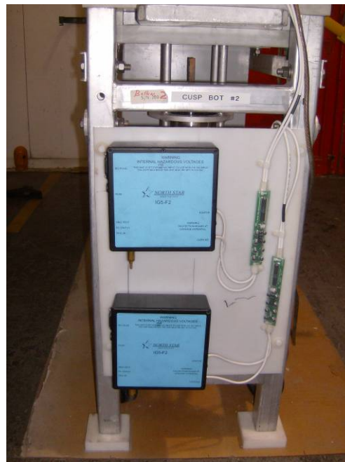
Figure 34. (a) Two 1.5 mF Cusp bank modules stacked on top of each other; (b) ignitron trigger units
