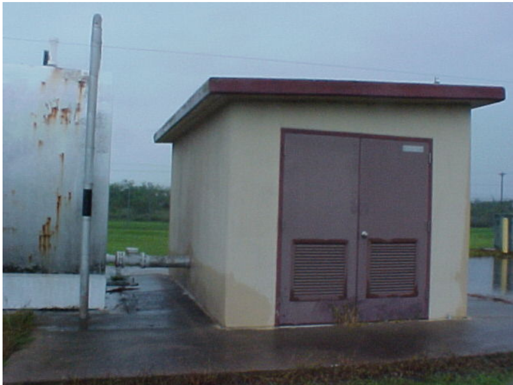
Photograph 12: Building T-22—Water Tank and Pump Storage Building
