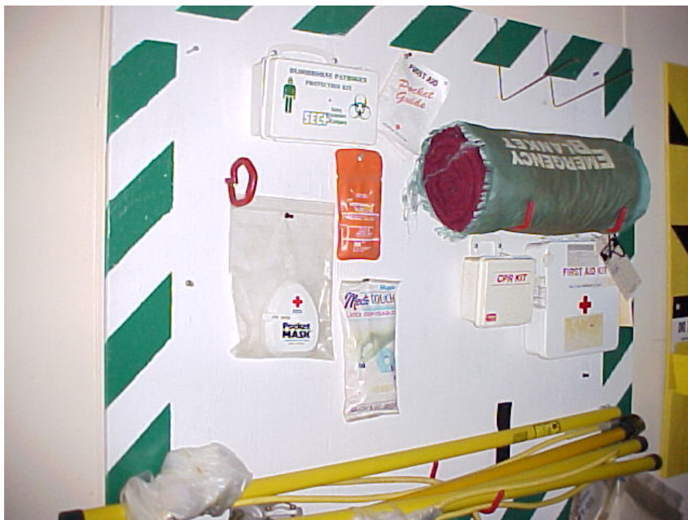
Photograph 41: First aid supplies found in Operations Building.
