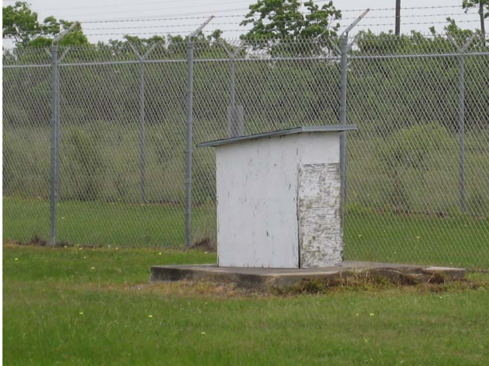
Photograph 11: Onsite water well with a depth of 685 feet. This well is located in the northeast corner of the site and produces water at 60 gallons per minute (gpm).
