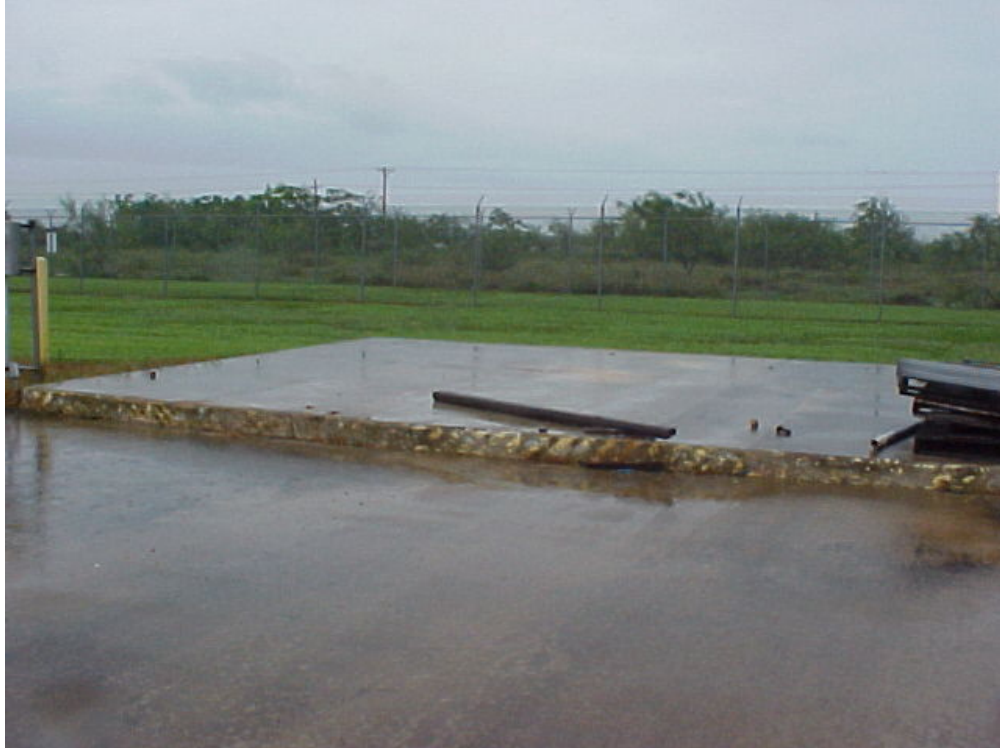
Photograph 49: Concrete pad with nothing on it.
