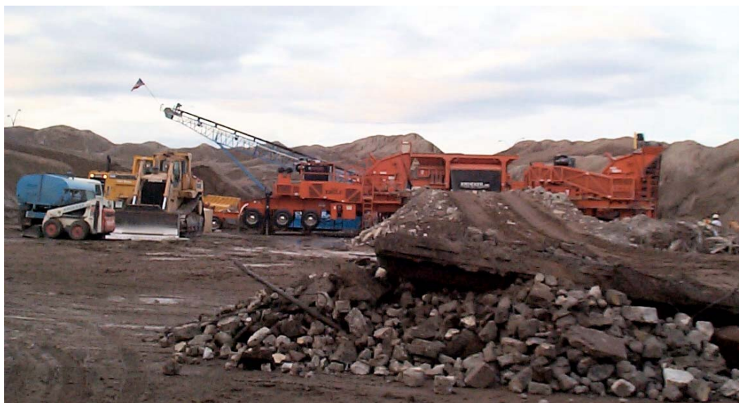
Figure 1. Overview of crusher plant.
