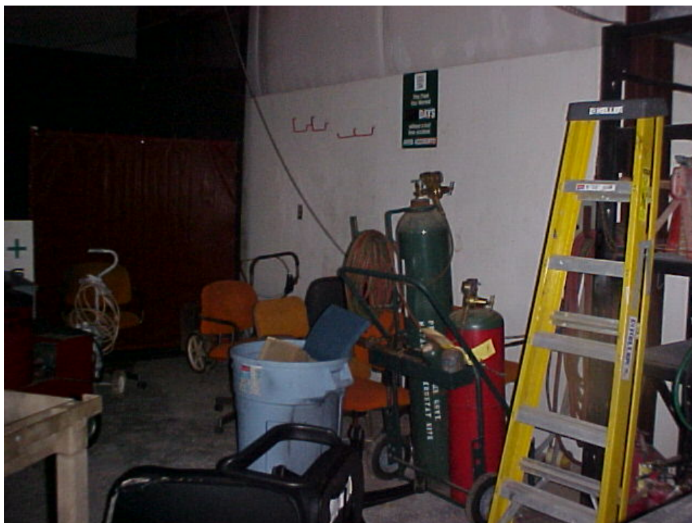
Photograph 22: Compressed oxygen tank and dissolved acetylene tank found in Building T-13.
