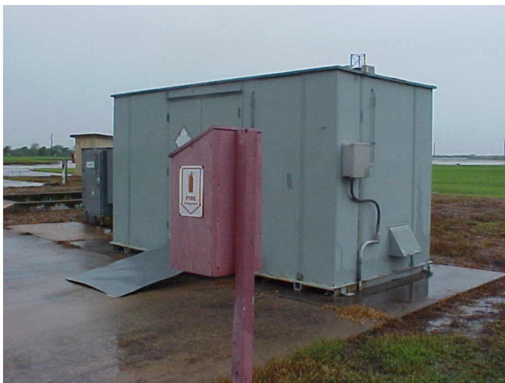
Photograph 14: Building T-16—Hazardous Materials Storage Building
