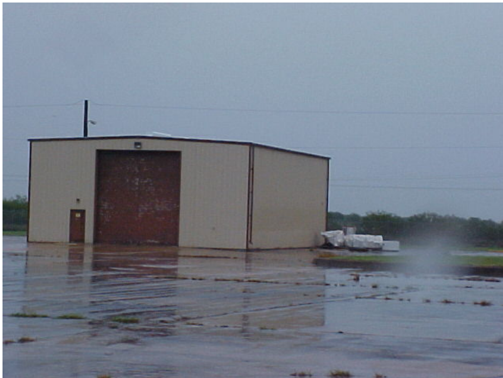
Photograph 16: Building T-04—Payload Service Building
