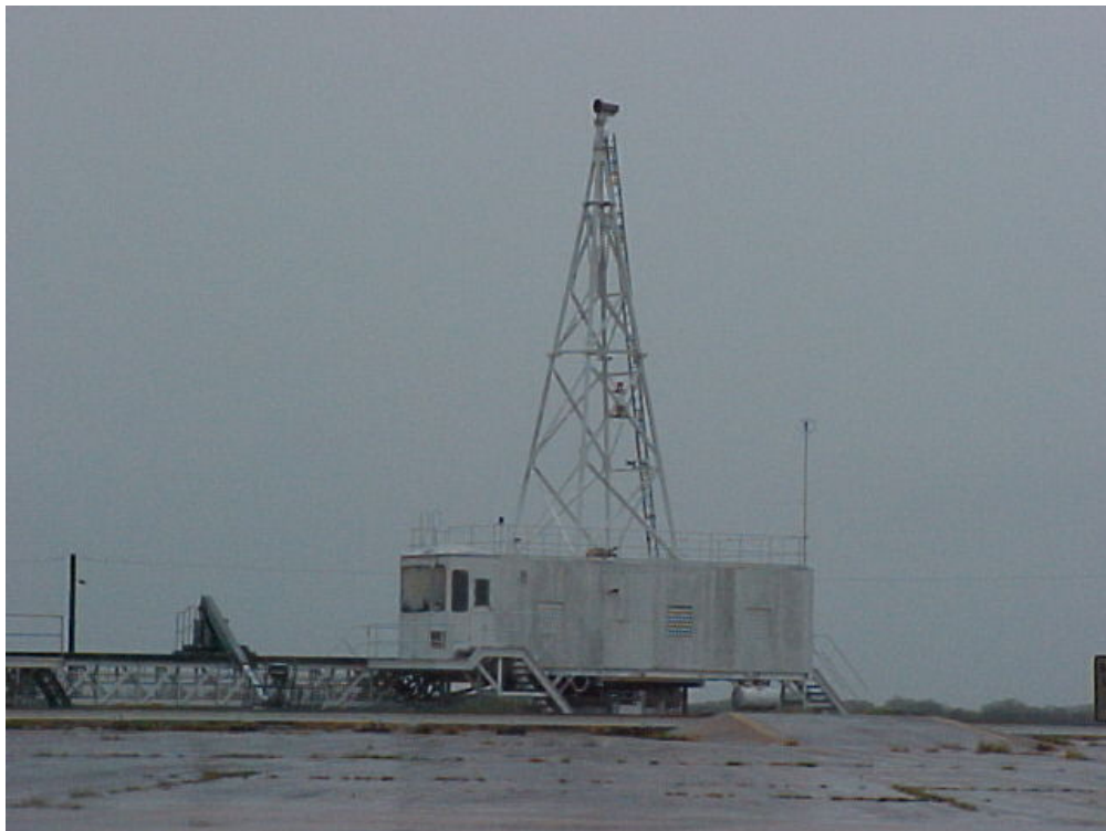
Photograph 50: The Aerostat pad and equipment at Matagorda TARS site.
