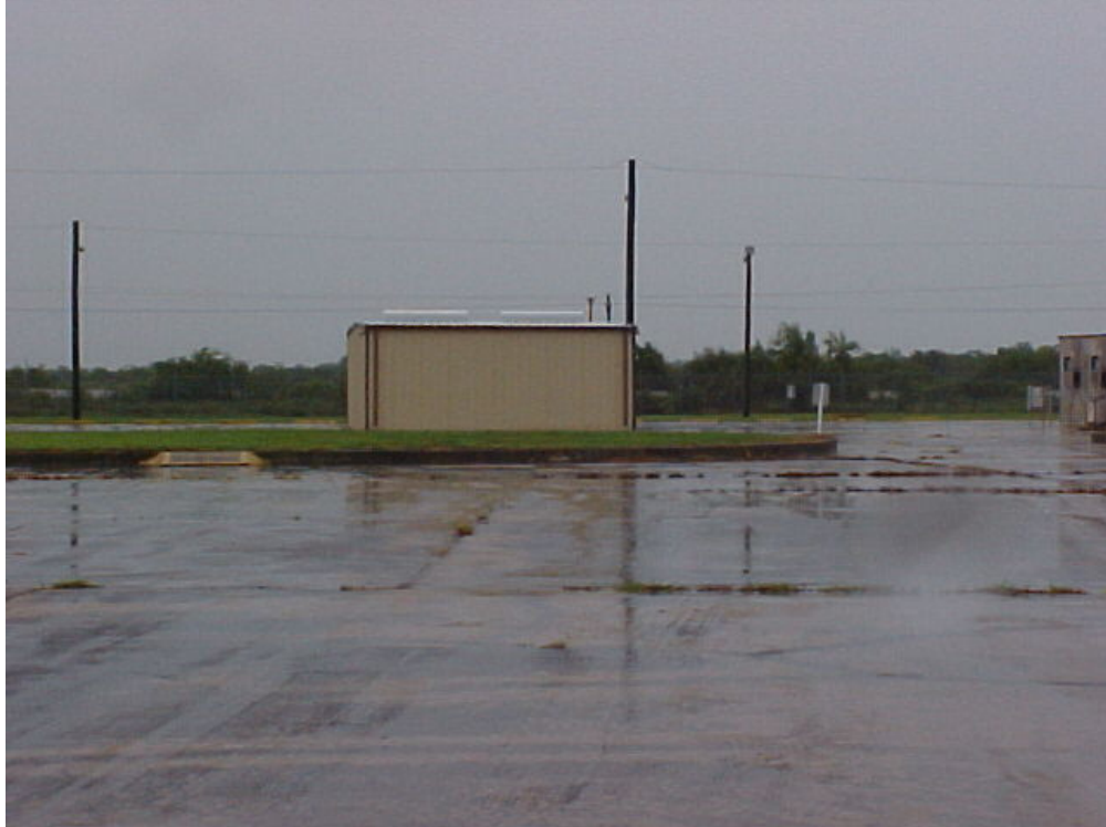
Photograph 35: Operations Building with the septic drainage field behind it.
