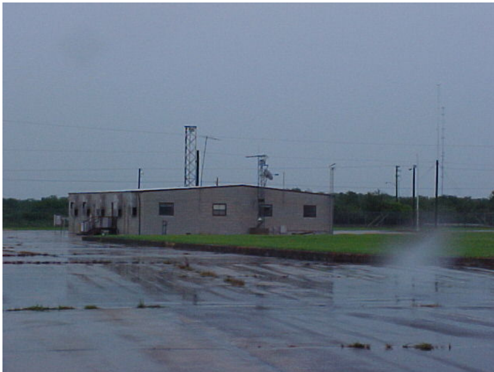
Photograph 36: View looking southeast showing the Operations Building.
