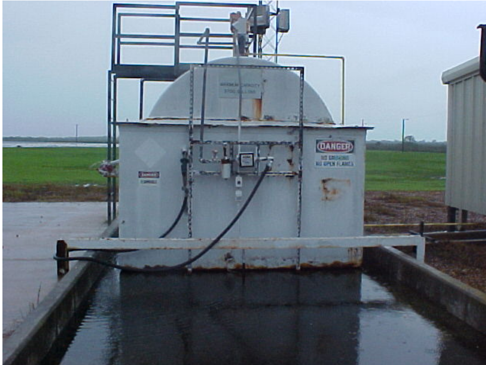
Photograph 1: 5,700-gallon aboveground storage tank (AST) at Matagorda TARS site. This AST is located just north of the Payload Service Building.
