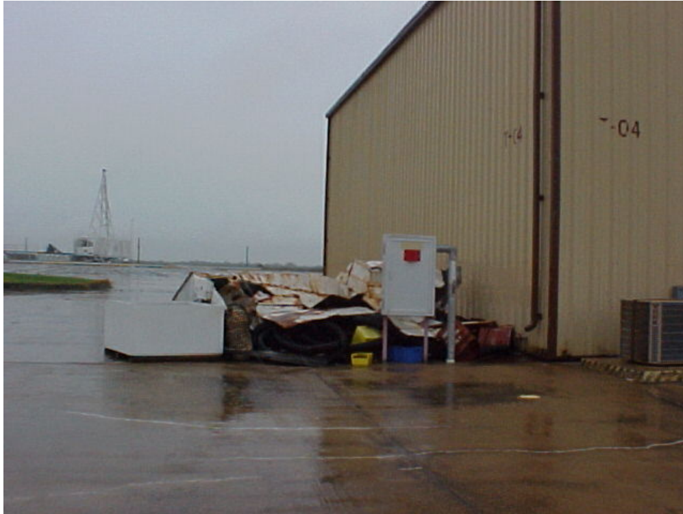
Photograph 17: Trash and debris next to Building T-04.
