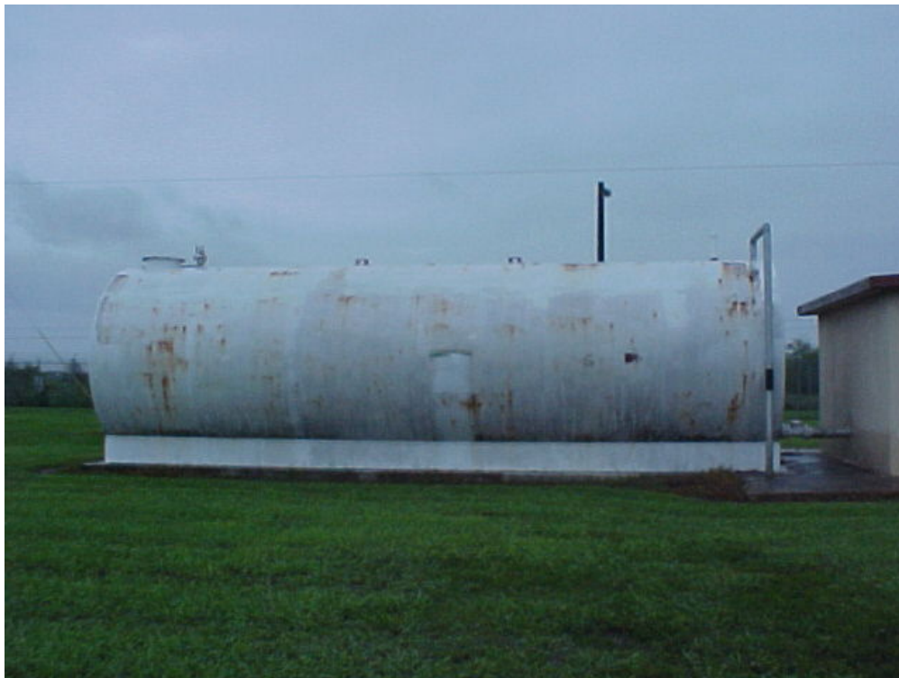
Photograph 8: 20,000-gallon water tank at Matagorda TARS site. This water tank is located on the northern portion of the site directly north of the Water Tank and Pump Storage Building.
