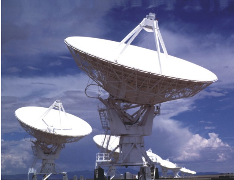
The Very Large Array, located near Socorro, New Mexico, consist of 27 radio antennas that are each 25 meters (82 feet) in diameter. It is the most scientifically productive ground-based telescope in the history of astronomy. (Photo courtesy of the National Radio Astronomy Observatory/Associated Universities, Inc.)
