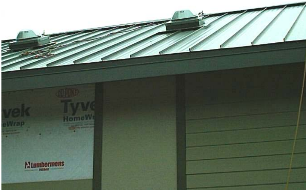
Figure 18. Standing seam metal roofing in place.
