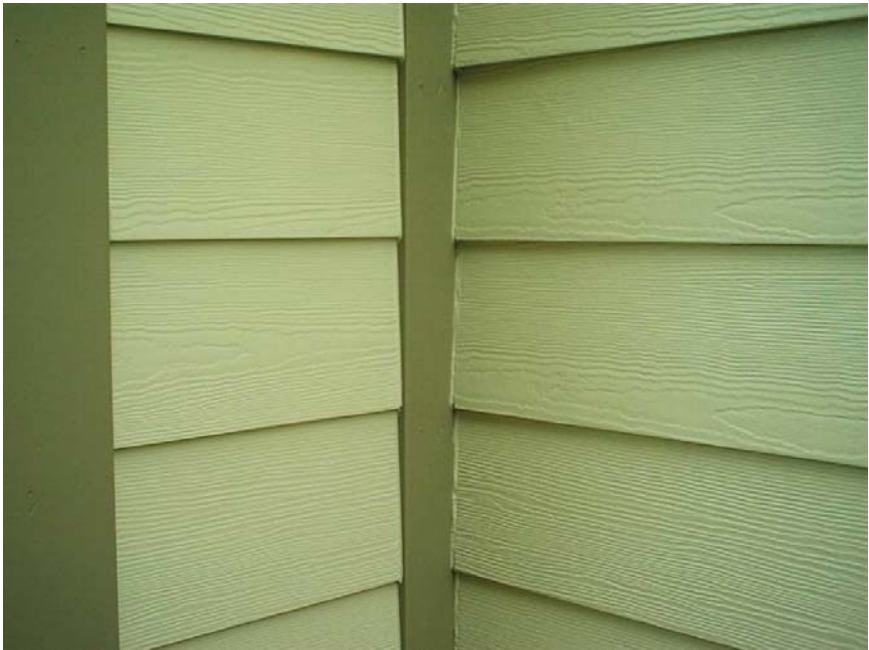
Figure 17. Hardieplank siding detail.
