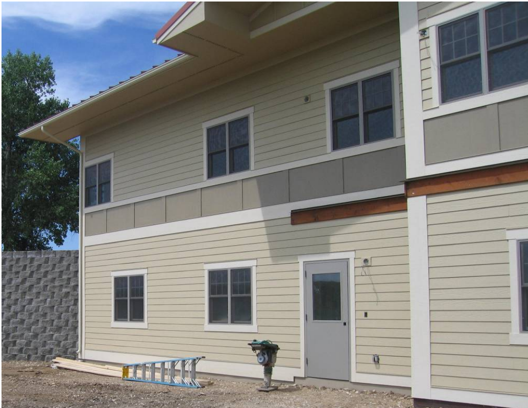
Figure 7. Example of Hardiepanel ship-lapped siding.
