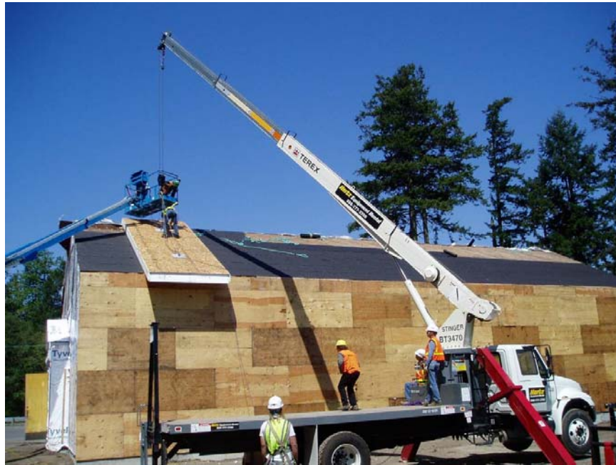
Figure 15. SIPS panel being placed.
