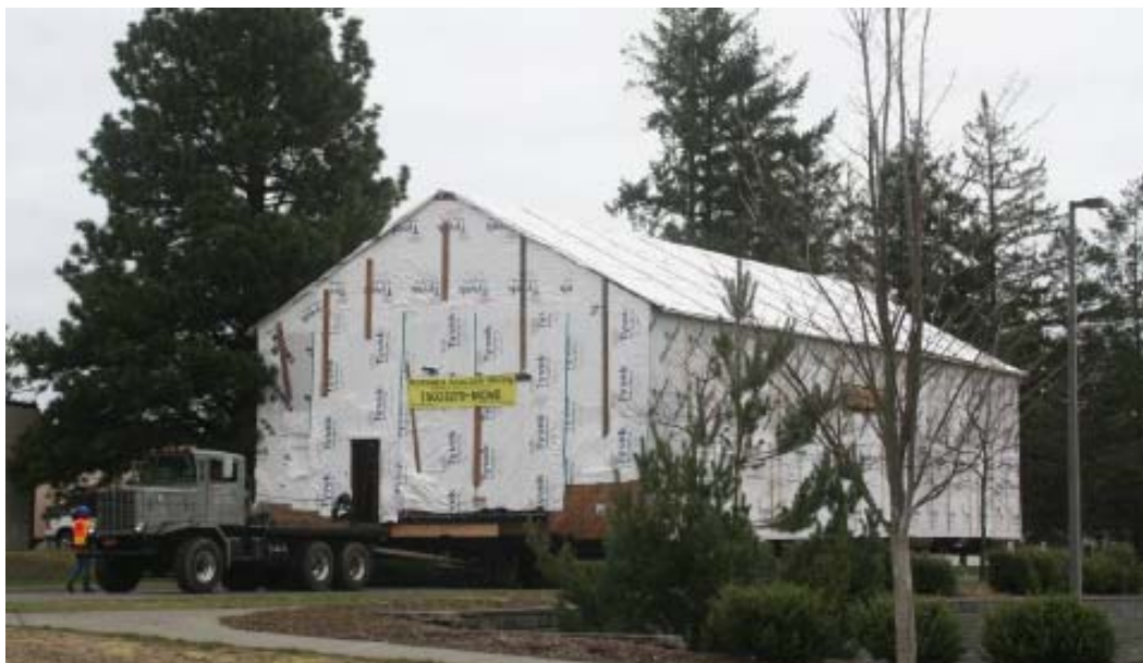
Figure 9. North Fort Chapel in transit to new location.
