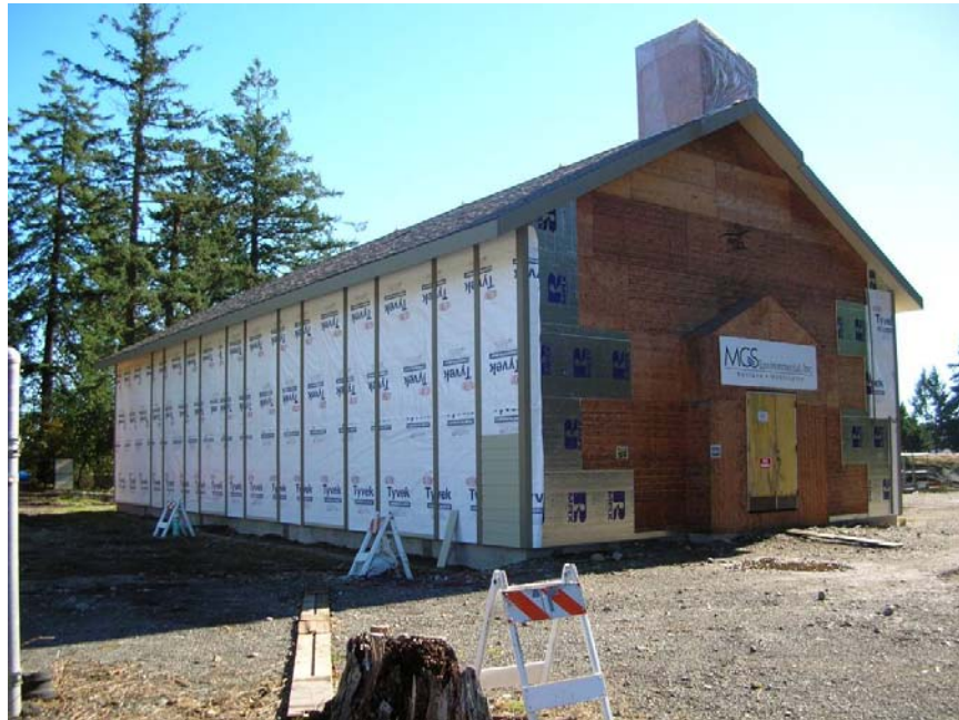
Figure 14. External insulation and air barrier in place.
