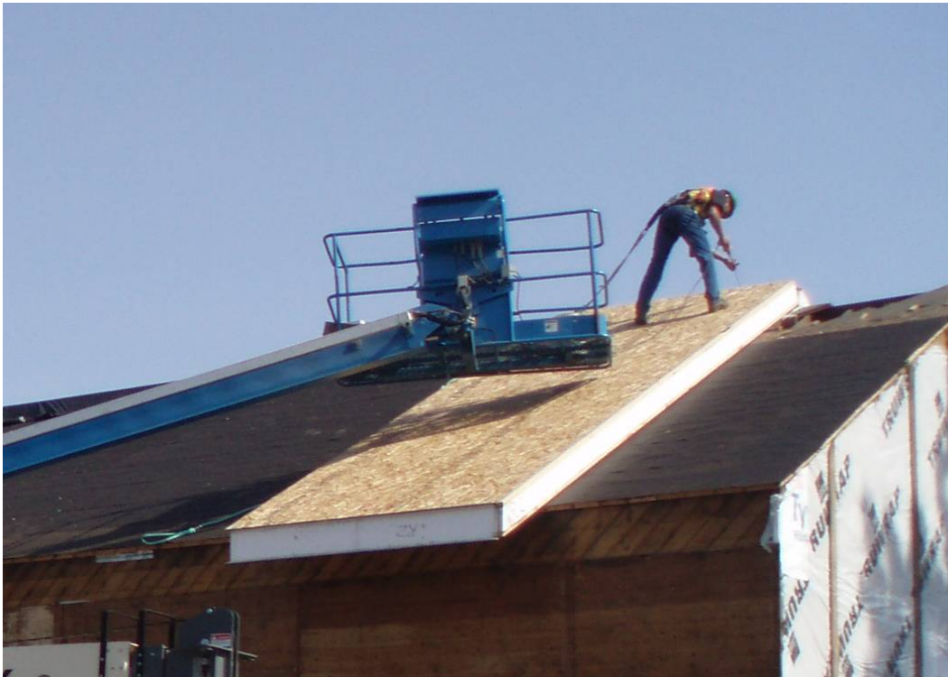
Figure 8. Sandwich-type SIPS panel being attached to roof.
