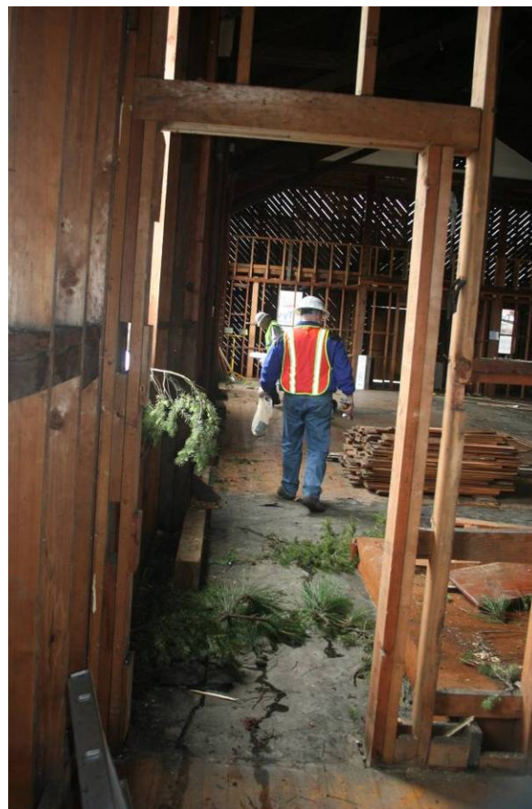
Figure 5. The relocated building's interior.
