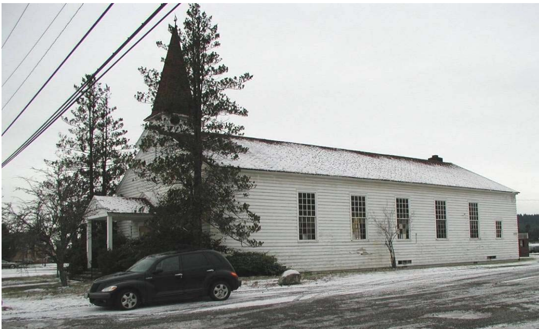
Figure 1. The existing chapel building before relocation.
