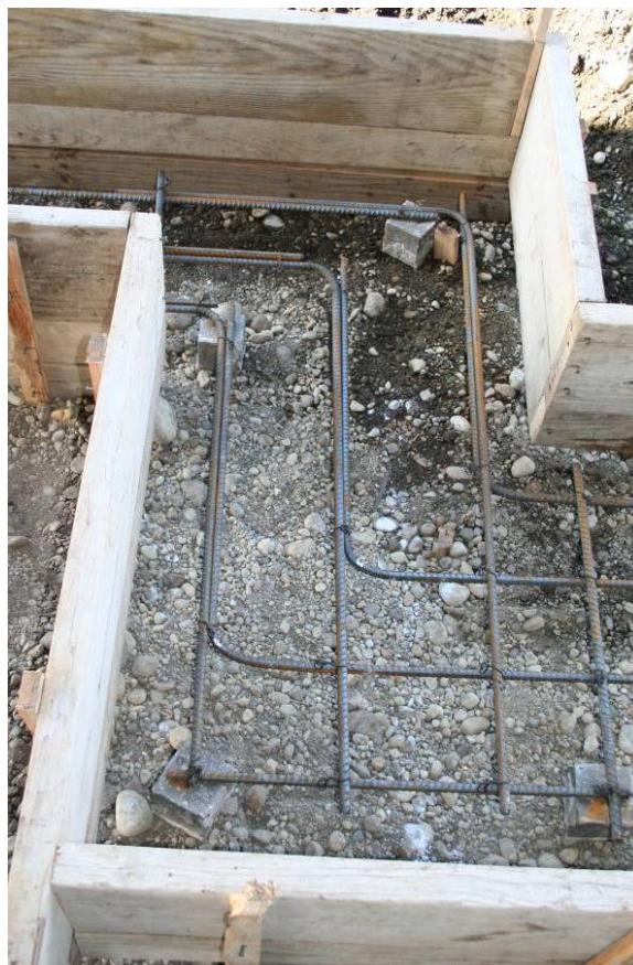
Figure 11. Footing forms and reinforcement bars under the building.
