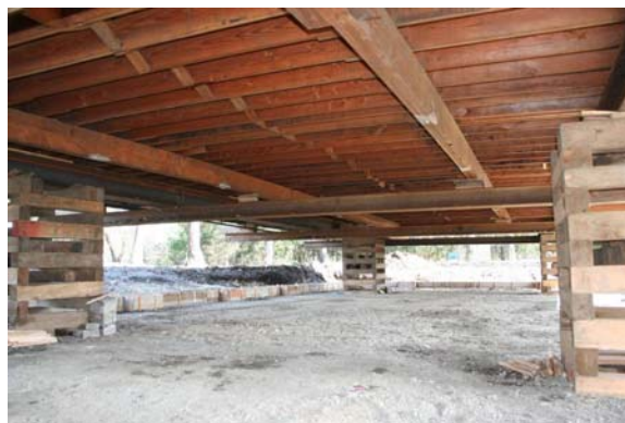
Figure 10. Underside of the building in place, supported by cribbing.
