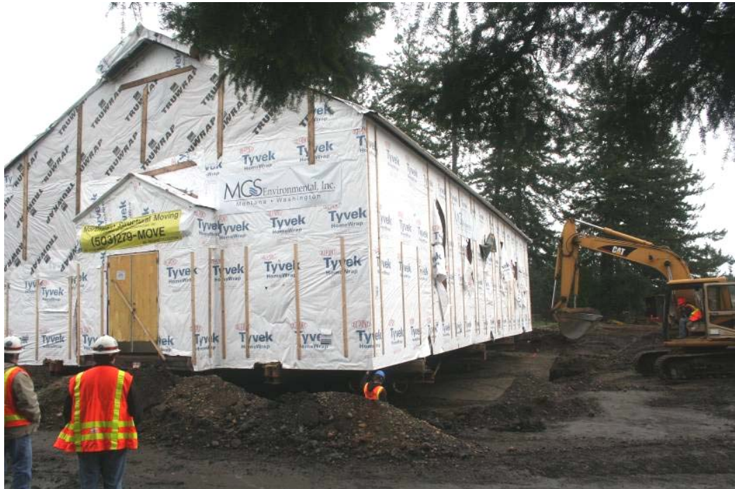
Figure 4. The relocated building's exterior.
