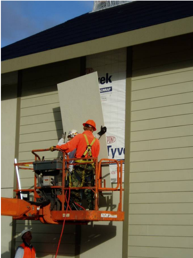
Figure 16. Installation of Hardieplank siding.
