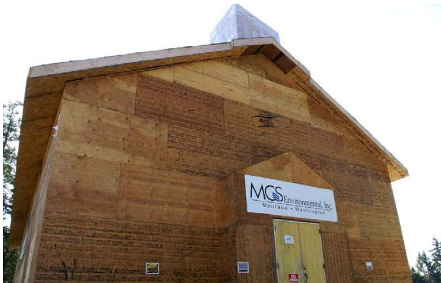
Figure 13. Salvaged plywood sheathing.
