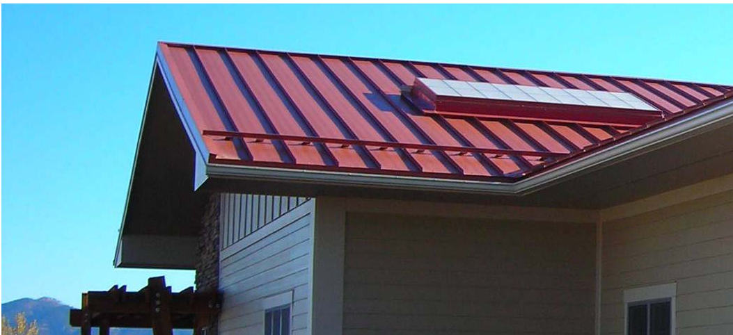
Figure 6. Example of standing-seam metal roof system.
