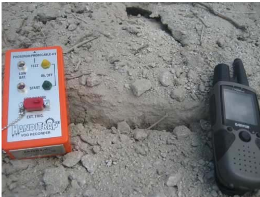
Figure 25. Largest crack generated by Shot 1.
