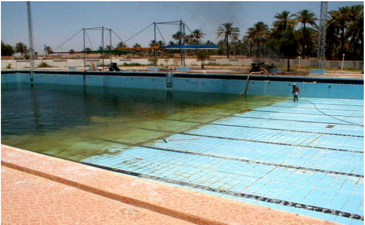
Photo 4. Al Hillah Olympic Swimming Pool
