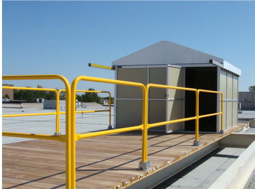
Figure 58: AFIT Roof Top Observatory
