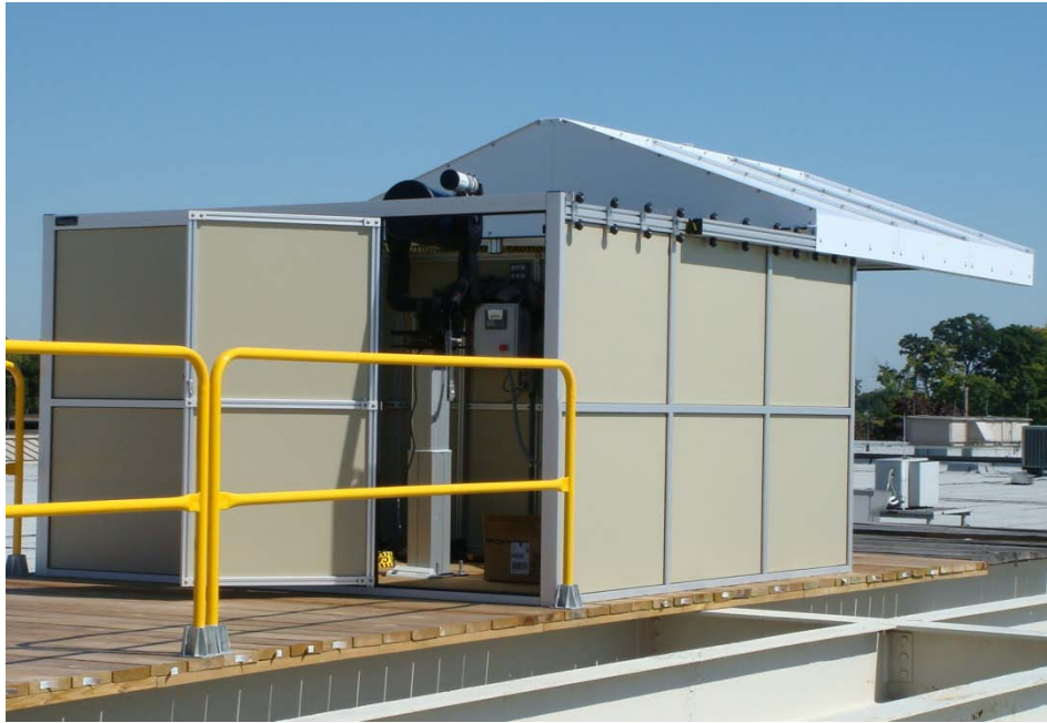
Figure 59: Observatory with Roof Open and Pier Actuated
