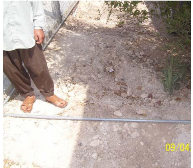
Site Photo 2. Water supply to guard house not buried (Courtesy of GRC)
