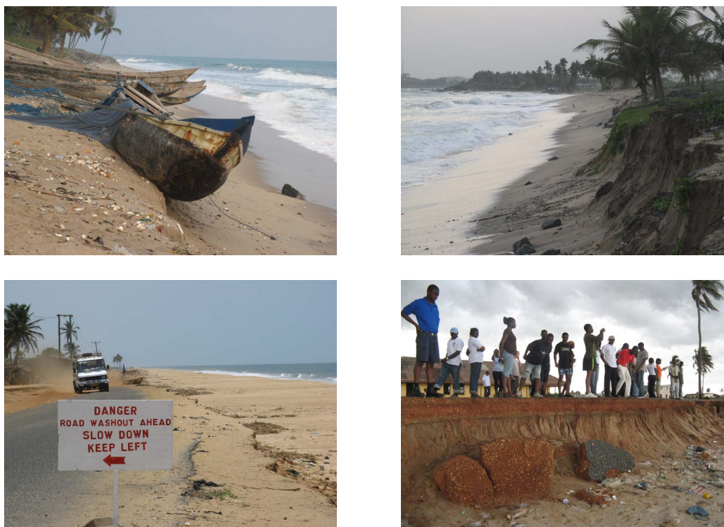
Figure 1. Active erosion at Ada (left bottom), Anyanwi (right bottom), and Accra (top panels) showing the effects of rapid beach erosion threatening major coastal roadways in the region.
