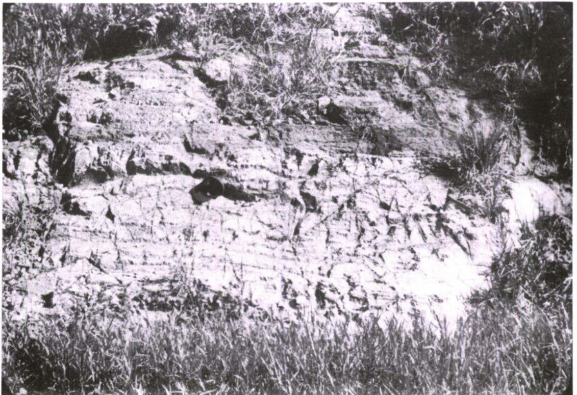
B. Unit No. 8 Weathered andesitic conglomerate and breccia. Cut along west side of Cross-Island Highway, district of Papago, east- central Saipan.
