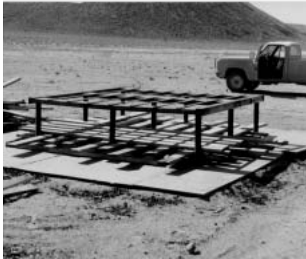
FIGURE 4. CONSTRUCTION OF TEST STANDS
