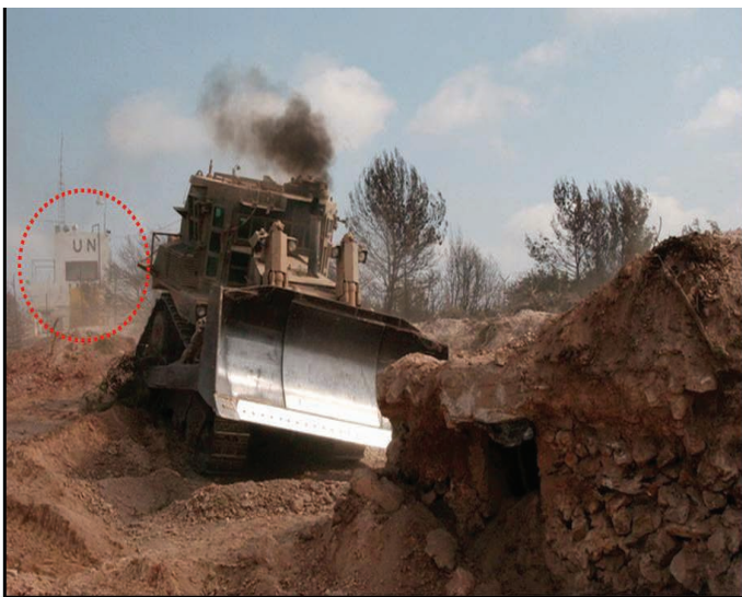
Uncovering a Hezbollah bunker adjacent to UN post
