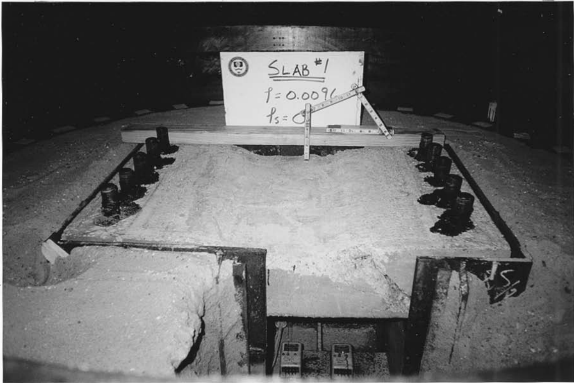
Figure 17. Posttest View of Slab No. 1
