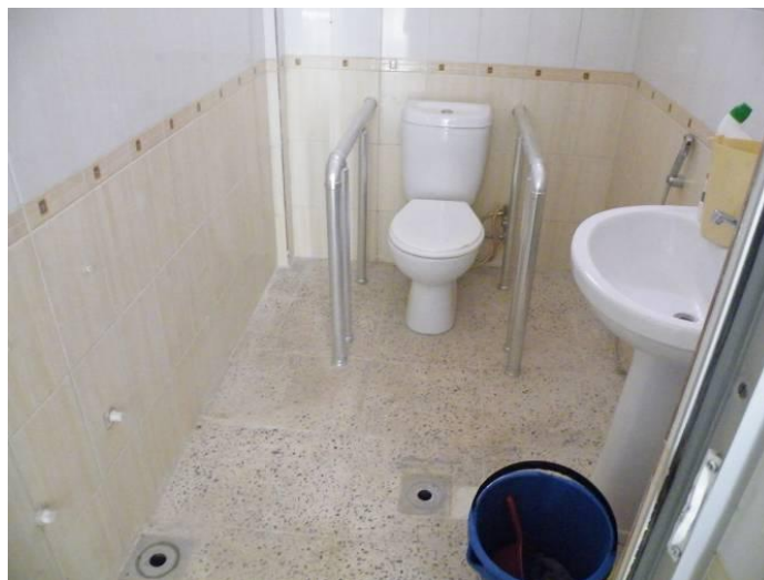
Site Photo 10. Accessible restroom
