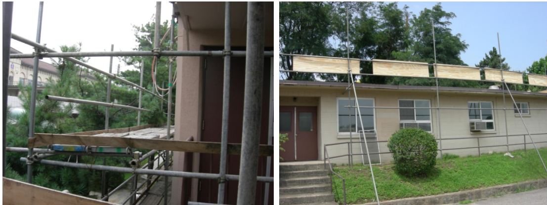
Figure 1. Scaffolding Around a Building Figure 2. Fall Protection for Roof Work
