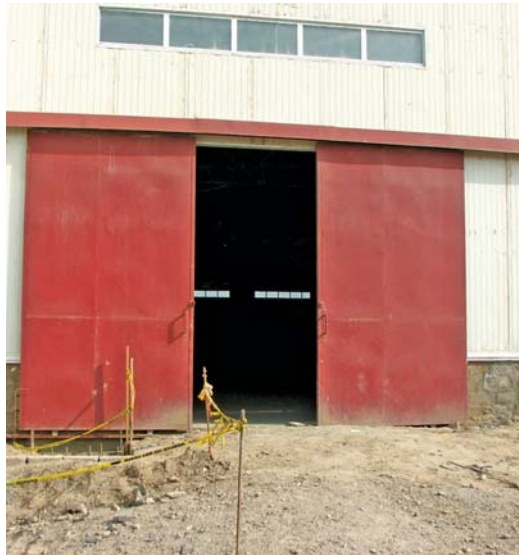
Entry door at the Abu Ghraib Dairy.
