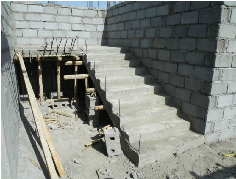
Site Photo 13. Reinforced concrete stairs
