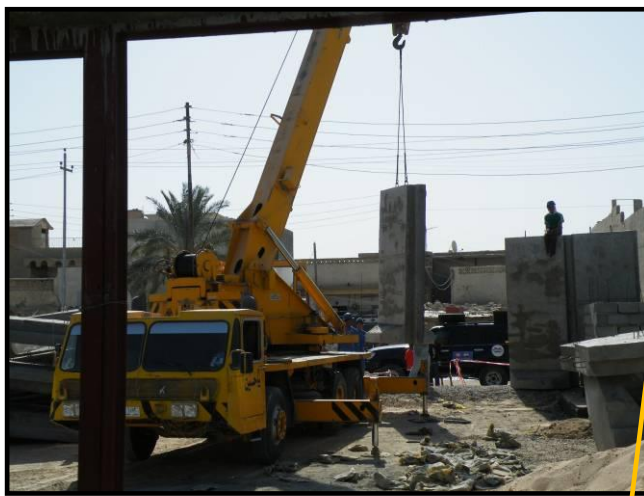
Site Photo 3. T-wall installation
