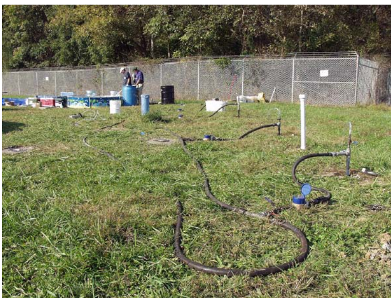
Figure 3. Injection of EOS ® to form the permeable reactive barrier.
