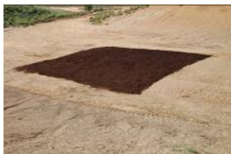
Figure 12. Photographs showing application of the PMSO material to Bay 1.
