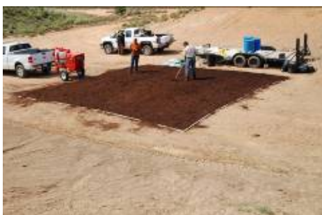
Figure 12. Photographs showing application of the PMSO material to Bay 1.
