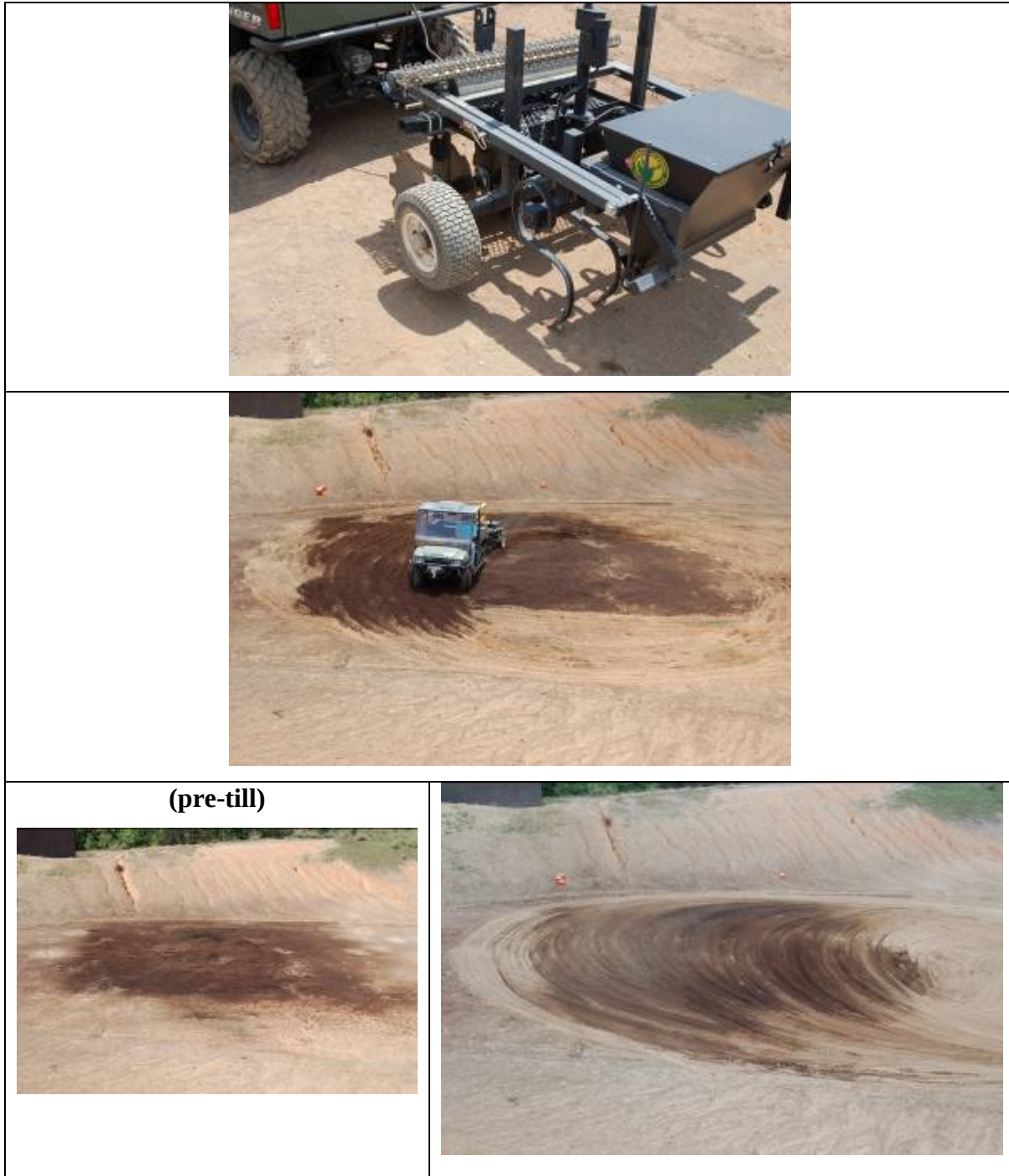
Figure 5.5-5. Photographs showing the PMSO layer being tilled into the soil in Bay 1.
