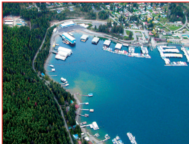
The Acoustic Research Detachment, built on the shores of Lake Pend Oreille, provides a deep, quiet body of water for testing, where an ocean-like environment is available without associated problems.
