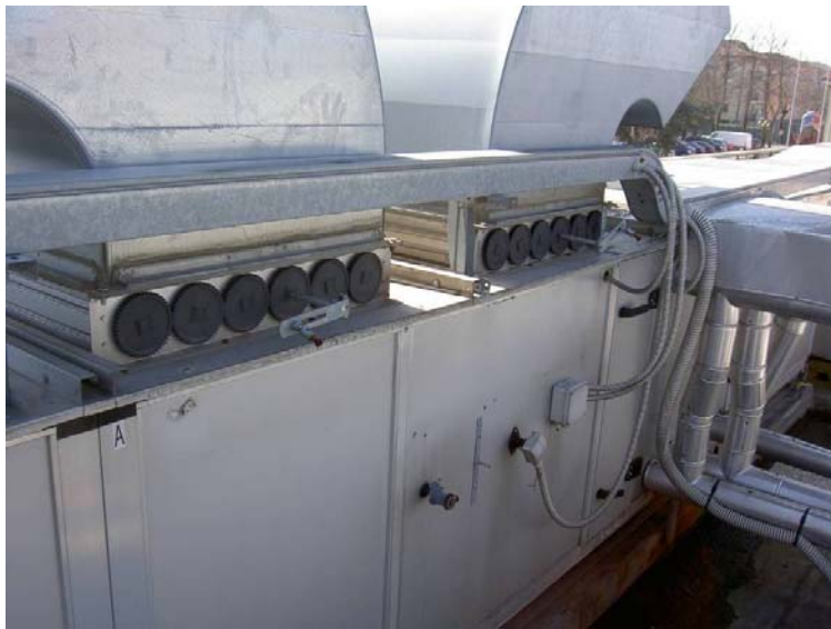
Figure 30. Nonfunctional damper control, missing metal link and the damper motor at Bldg 108.
