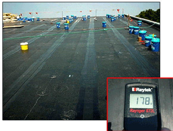
Figure 4. Roof before treatment, thermometer reads 178 °F at the roof surface on a hot summer afternoon.
