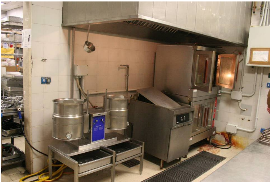
Figure 18. Typical kitchen hood with no extensions down or skirts at ends.
