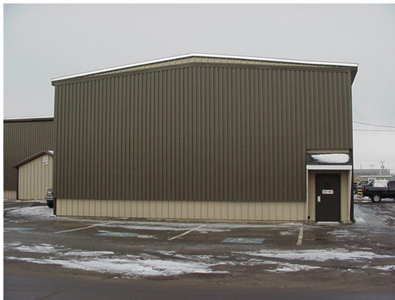
Figure 39. Example building with solar wall.
