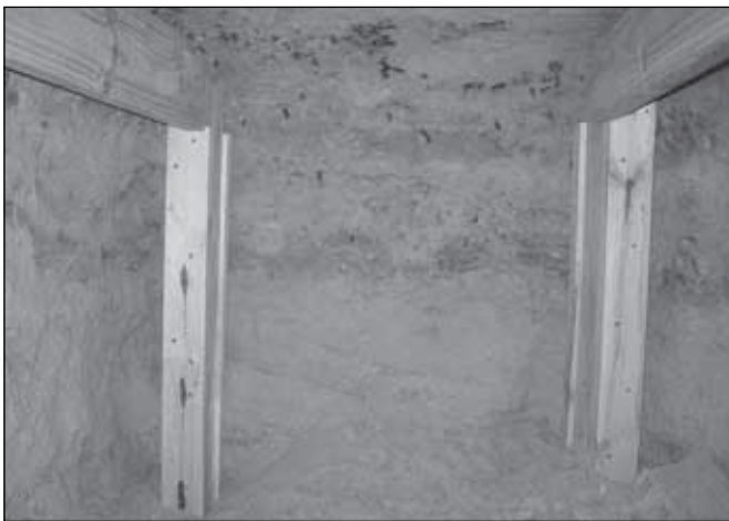
Figure 3. Black mineral concretions at the tunnel face. Striking these minerals makes a distinctive noise.
