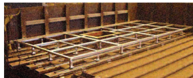
Aluminum False Deck Grid and Foundation
