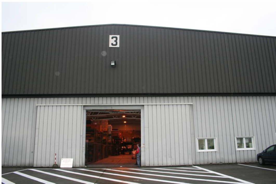
Figure 8. Truck Door in Bldg 2003 with opening at bottom.
