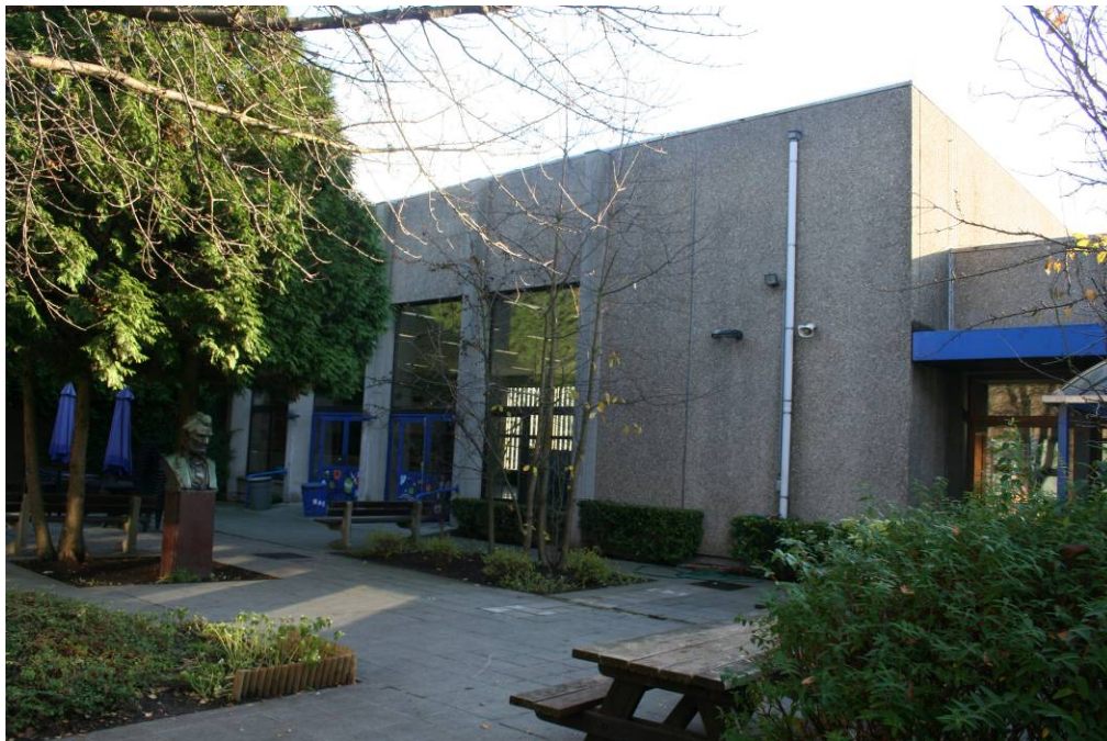
Figure 37. Double set of doors where new weatherstripping is needed.
