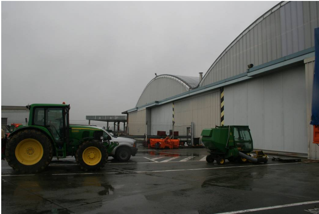
Figure 11. Southeastern wall of Bldg 2006 with two large vertical sections for solar collector.
