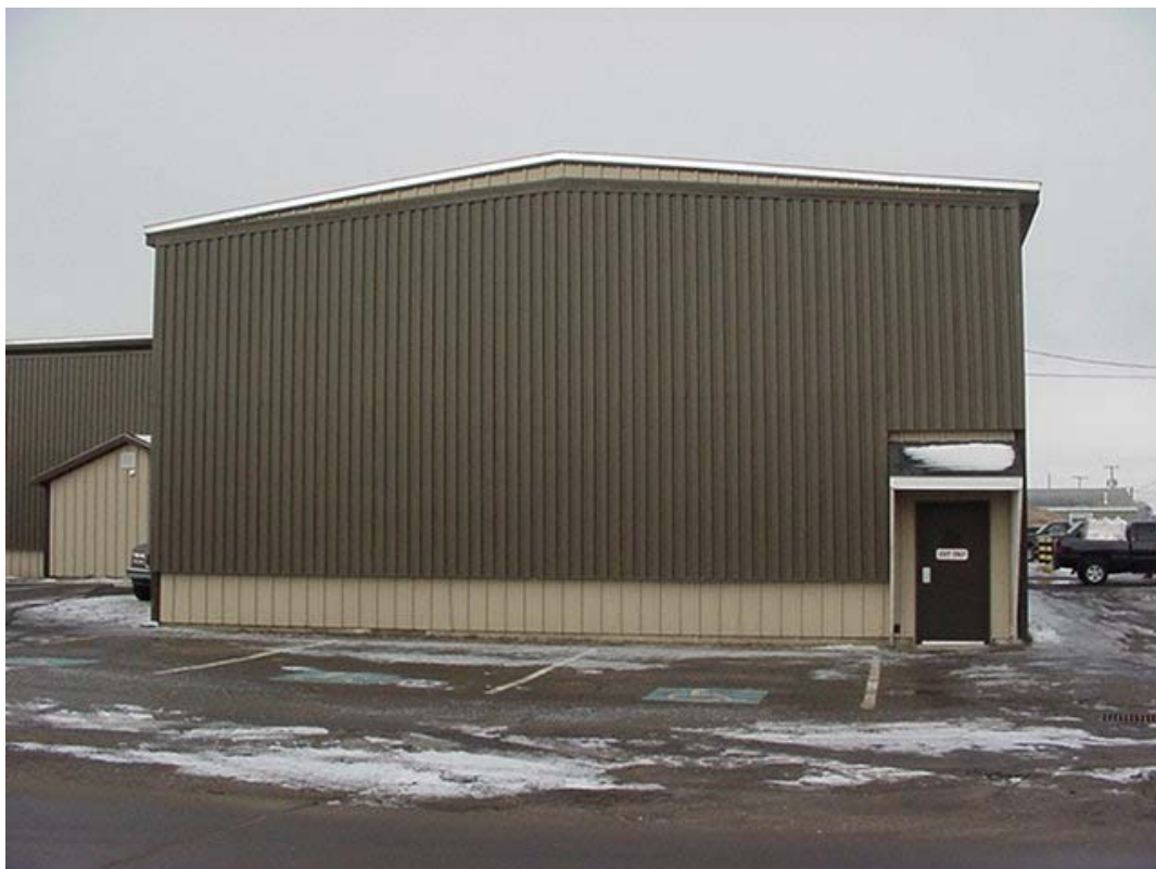
Figure 12. Building with solar wall.
