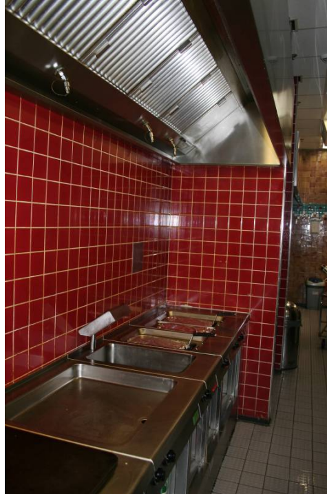
Figure 25. BBQ kitchen Hood that is good candidate for variable air flow.
