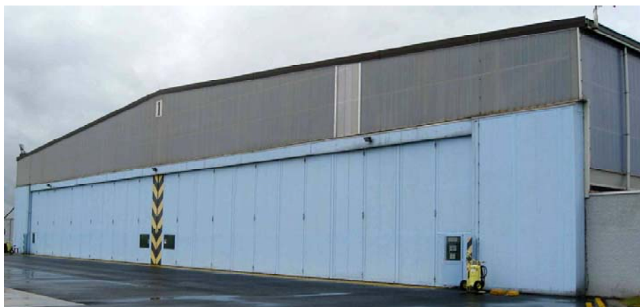
Figure 15. Hangar Bldg 1 at Chievres.
