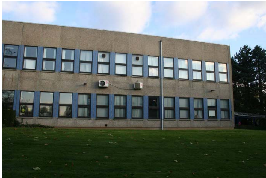
Figure 38. Condensers of classroom air-conditioner units.
