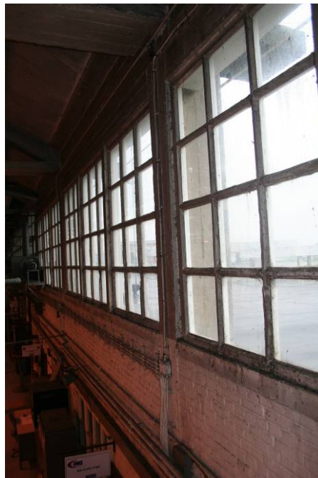
Figure 5. Inside of Bldg 2006 showing section of single pane windows.
