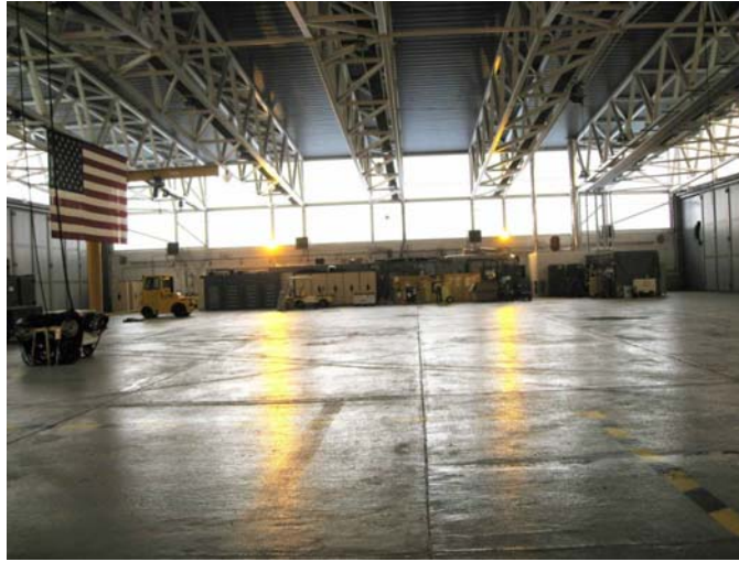
Figure 16. Inside of Hangar Bldg 2 at Chievres.
